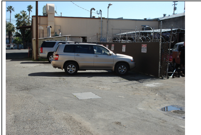
Photo 1. Rear of Halford's Cleaners building.
