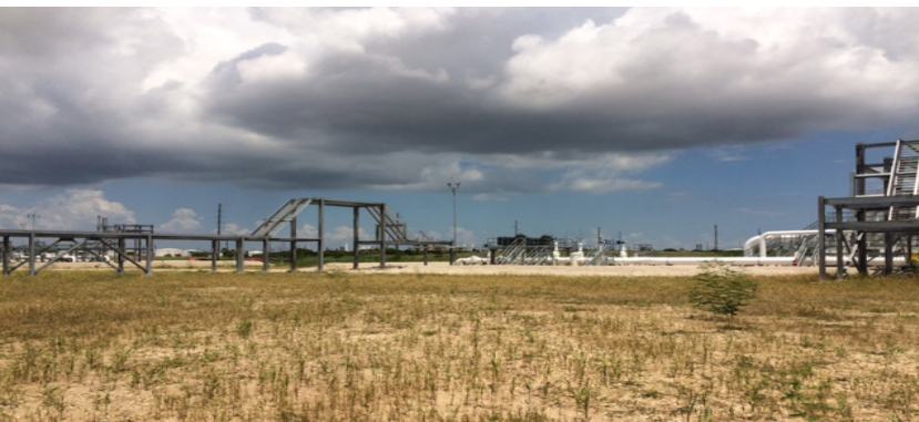
The bulk oil storage and transfer facility at the site. (Source: Genesis)
