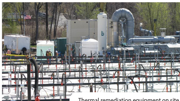
Thermal remediation equipment on site.
