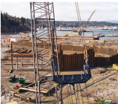
Installation of sheet piling.
