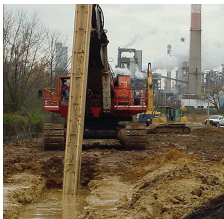
Excavation of a slurry wall trench.
