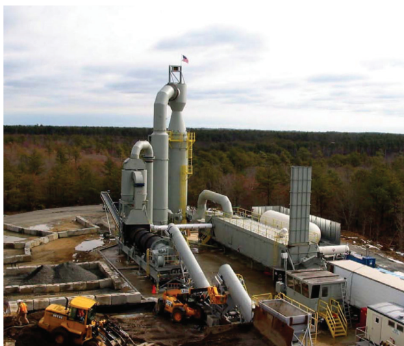
Onsite thermal desorber.
