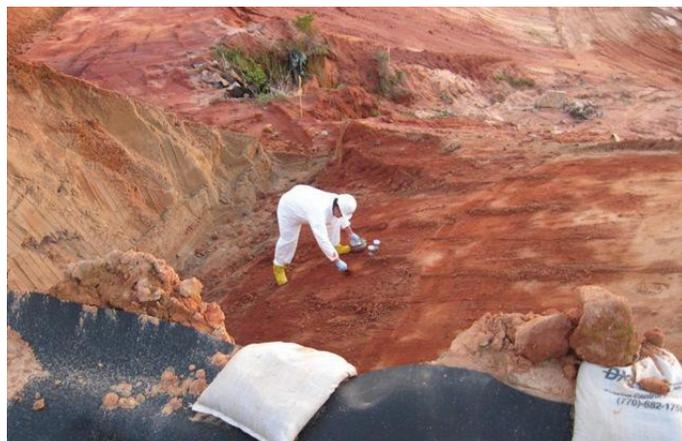
*Worker collects soil samples to confirm that soil left onsite is clean.*
