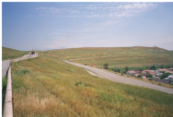
Spring grasses grow on the cap of a hazardous waste landfill.
