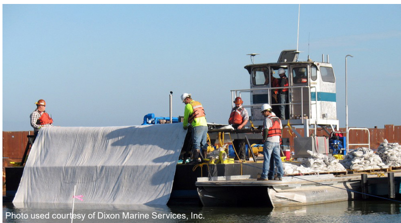
Placement of an amendment mat containing organoclay.
