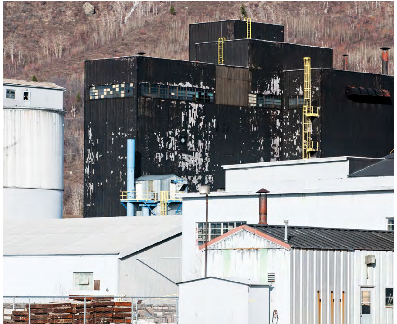
Buildings at the Columbia Falls Aluminum Company site. //Source: Flathead Beacon
