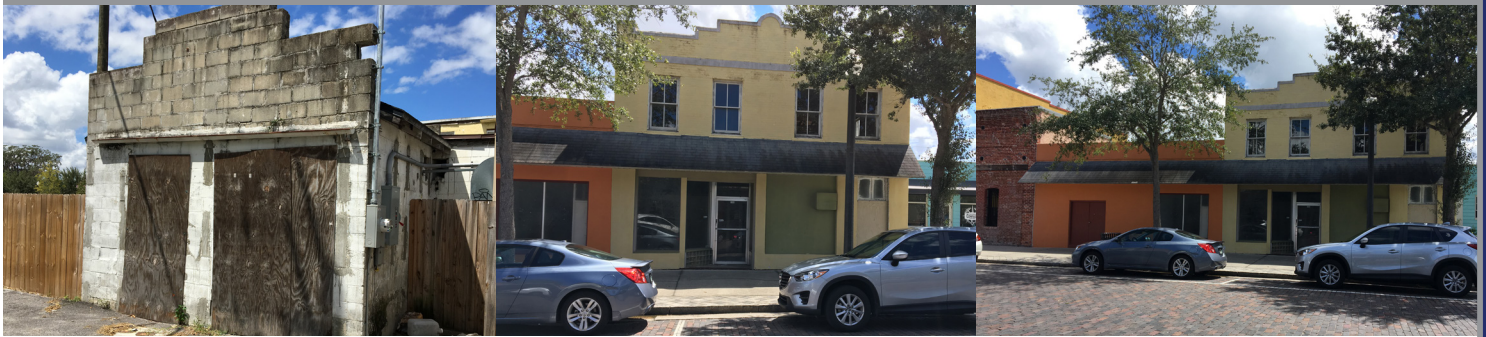
Images from left to right: Views of site buildings.
