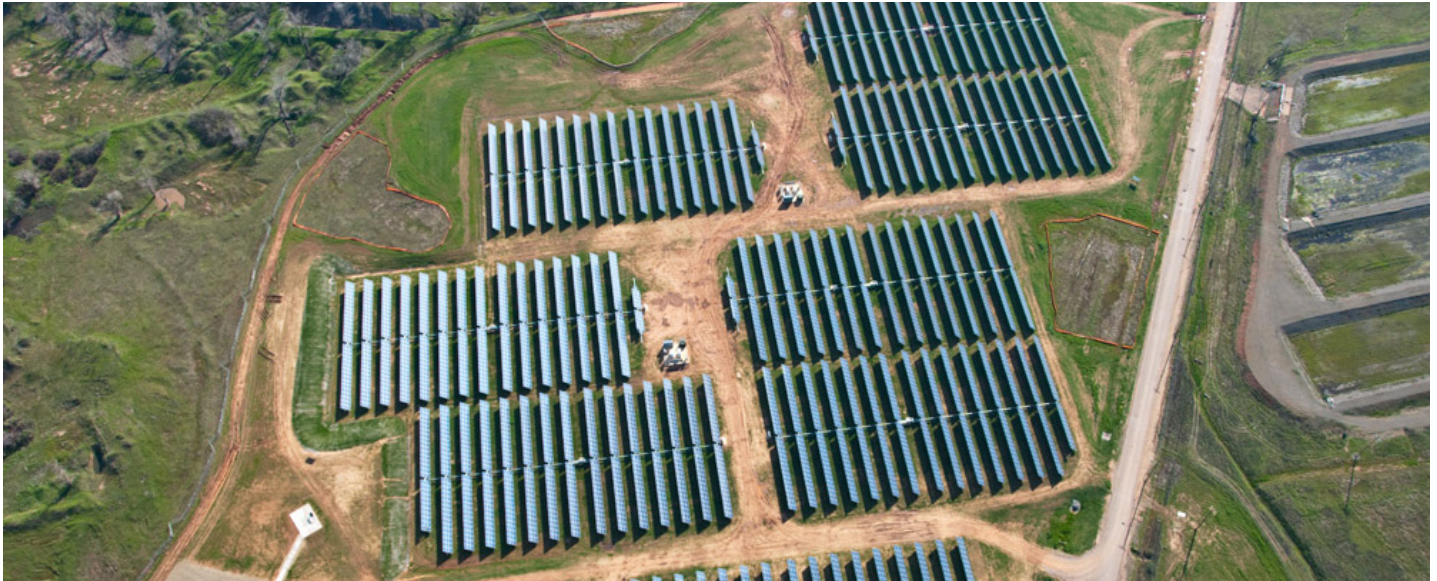
Aerial view of the site's solar facility.
