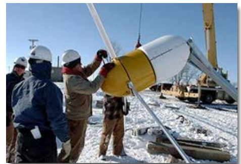
Figure 9. Installation of a wind turbine (Nebraska)
