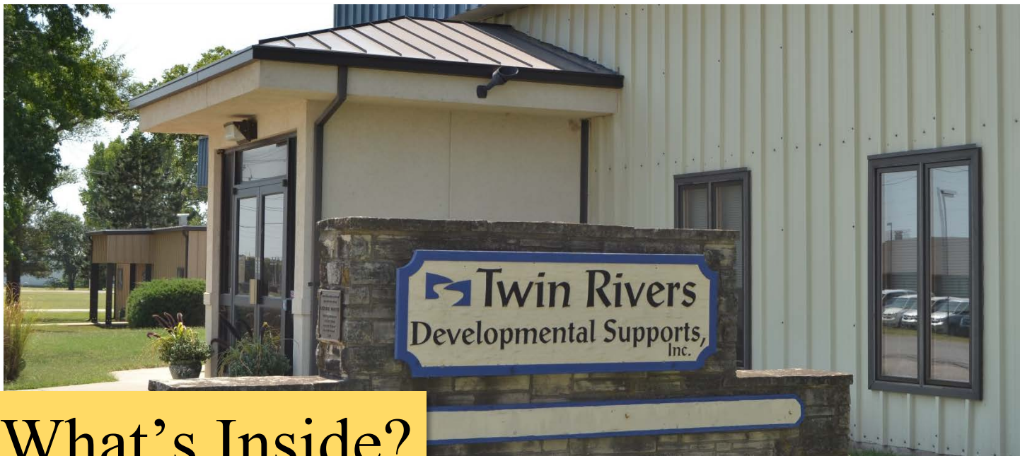
Figure 1. Strother Field Industrial Park site (Kansas)
