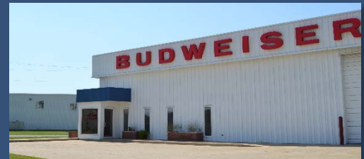
Figure 2. Ark Distributing (Budweiser) at Strother Field Industrial Park site (Kansas)
