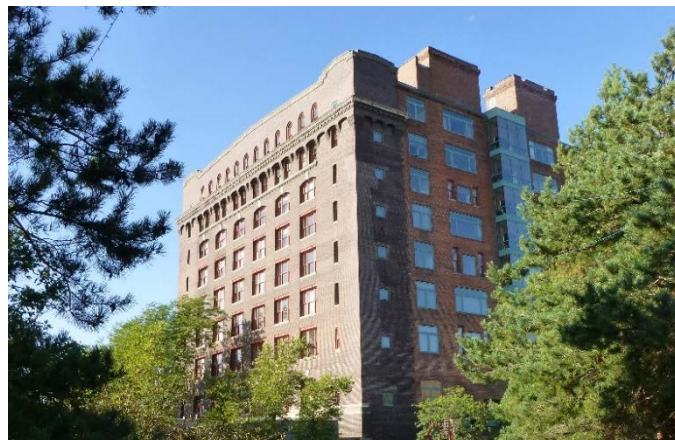
Figure 19. Residential apartment building at the Omaha Lead site (Nebraska)
