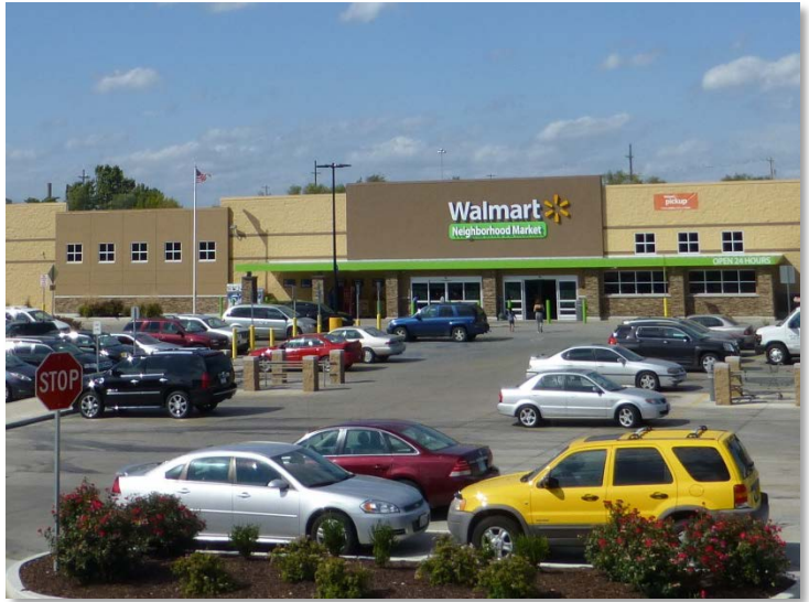
Figure 18. The new Walmart store at the Kansas City Structural Steel site (Kansas)
