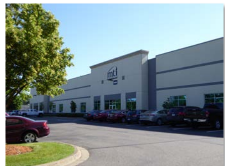
Figure 7: MTI Distributing's corporate headquarters.
