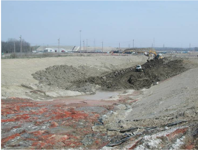
View to the east of sludges exposed in the Waste Pit 5 excavation with the On-Site Disposal Facility in the background (2004).
