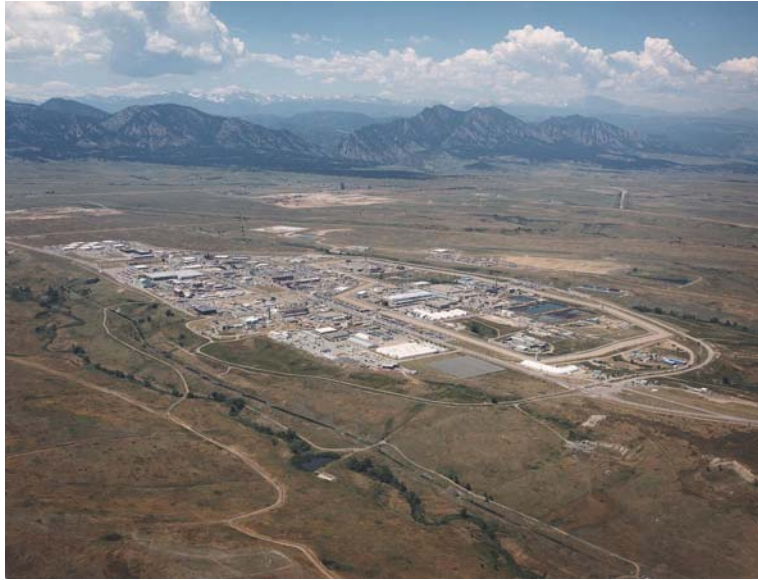
One of DOE's closure sites; view to the northwest.
