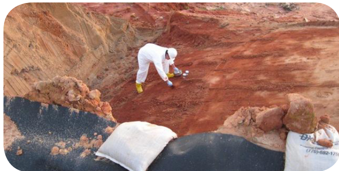
Worker collects soil samples to confirm that soil left onsite is clean.
