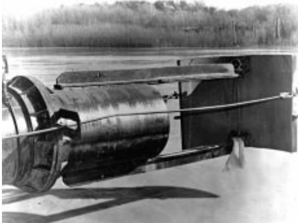
Figure 6. Spreader plate for hydraulic pipeline discharge
