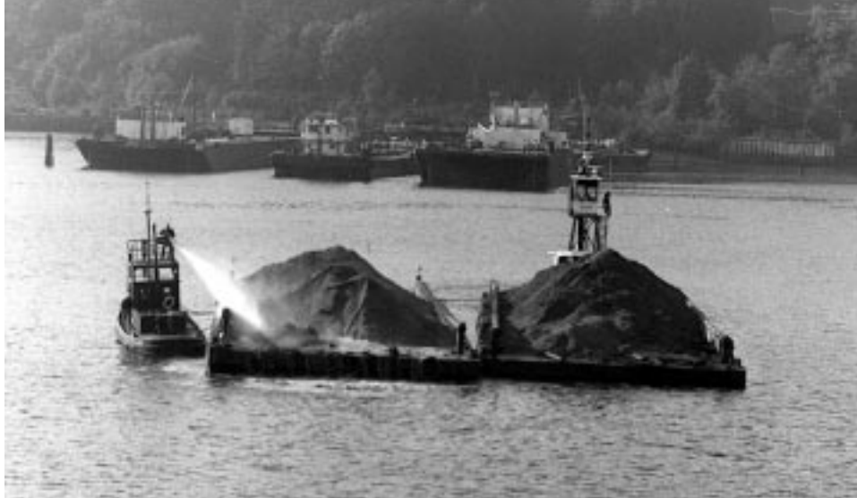
Figure 5. Pressure-hose washing method of placement
