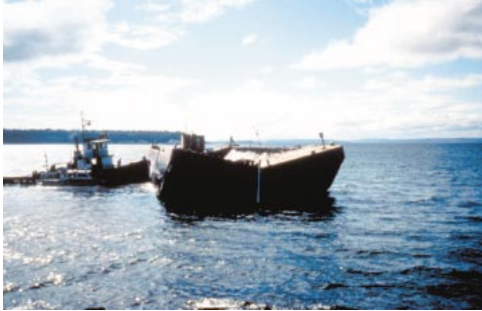
Figure 4. Spreading technique for capping by barge movement
