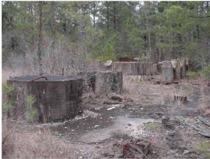
Photo 1 - South Tank Cradle
