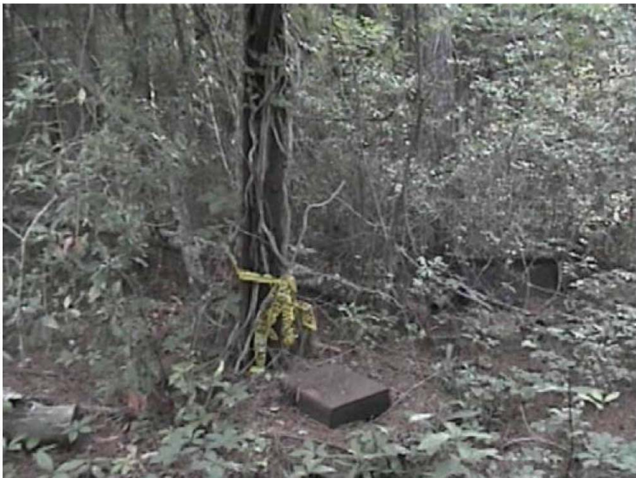
Photo 3 - Rusted rectangular box is covering a production well
