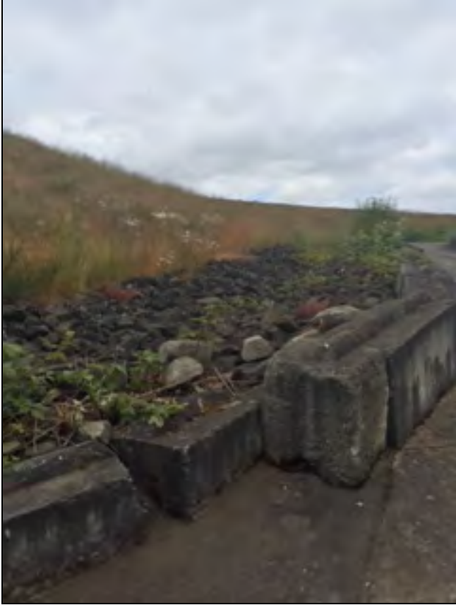
Photo 9. Vegetation growing in armored drainage channel between waste pile and access road.
