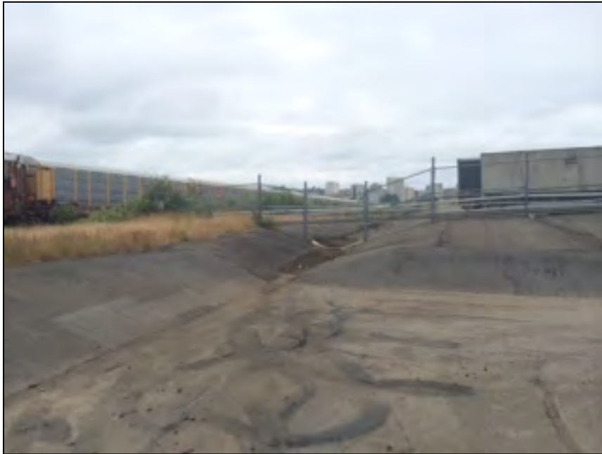
Photo 4. Drainage into Detention Basin 1
