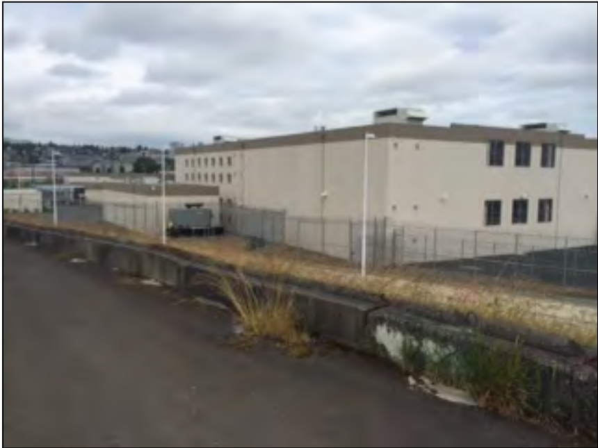
Photo 10. NW Detention Center Expansion from access road on top of waste pile.
