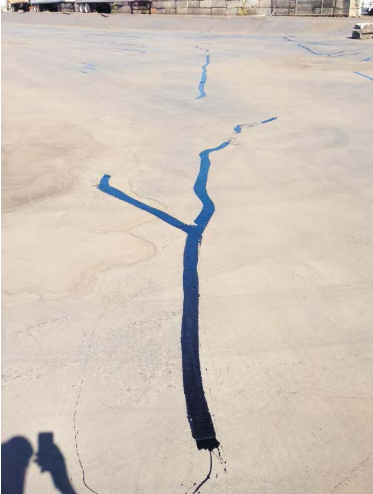
Figure 6-3. Photo of 2013 Asphalt Crack Repair in Detention Basin (Source: DOF 2014c)
