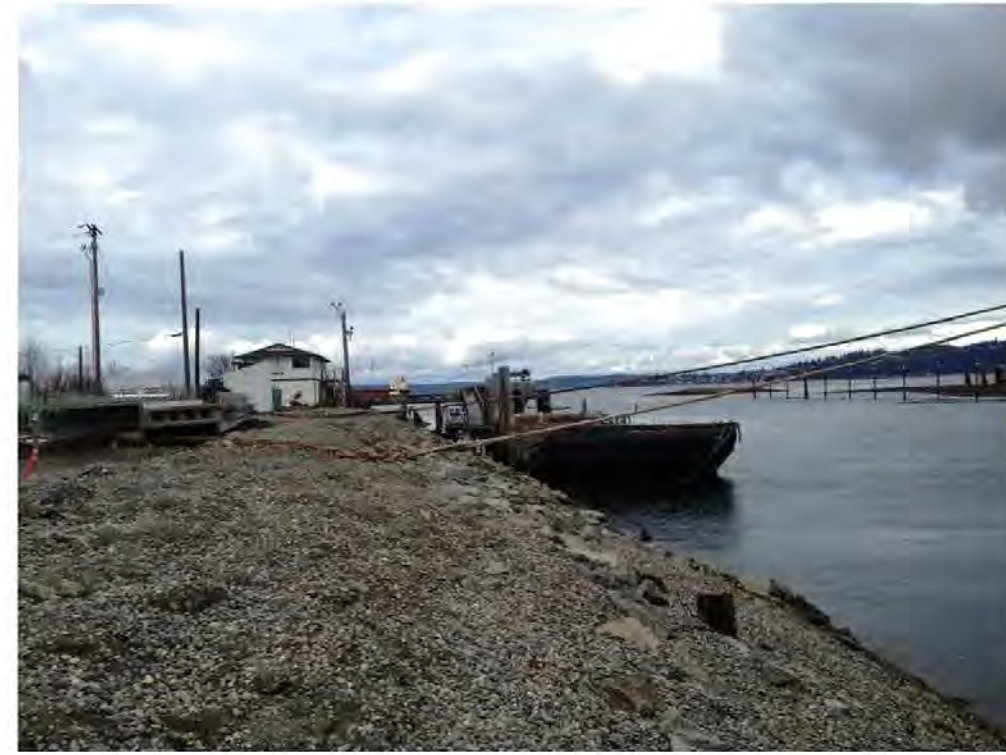
View from south shoreline looking north. (After)
