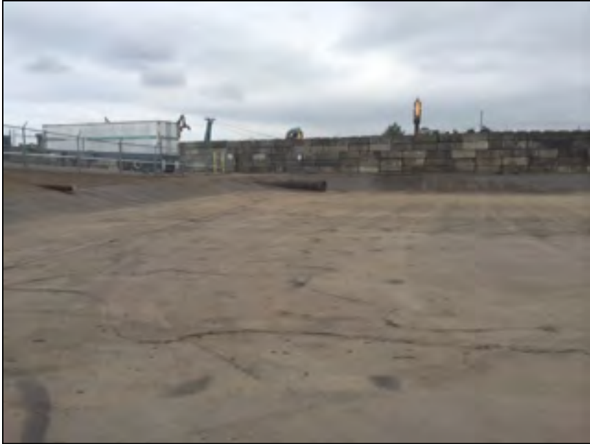
Photo 5. Drainage pipe into Detention Basin 1.
