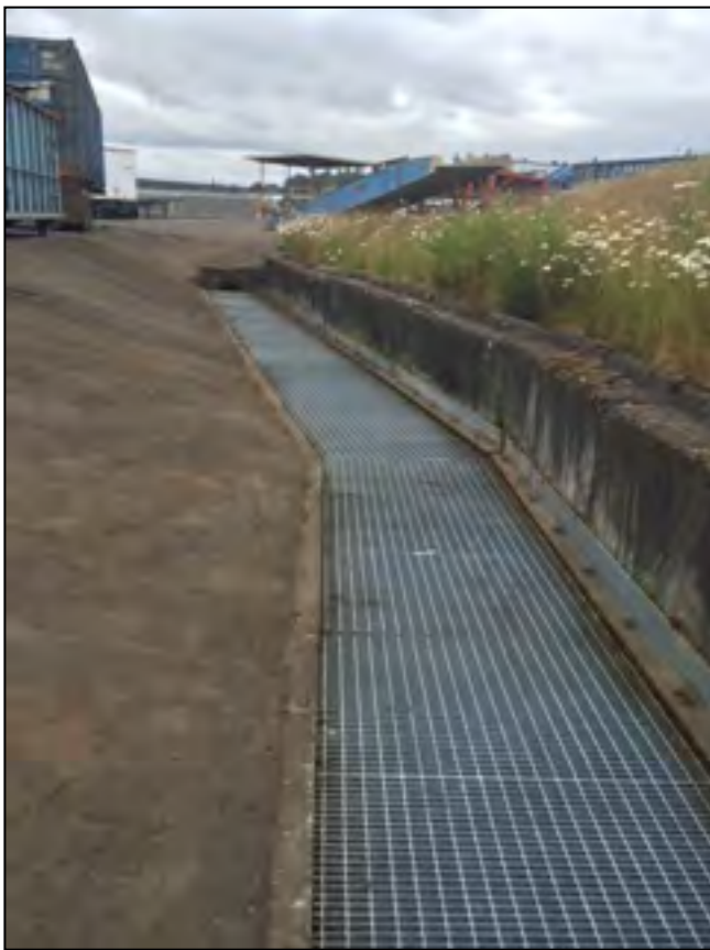
Photo 8. Perimeter drain clear grates.
