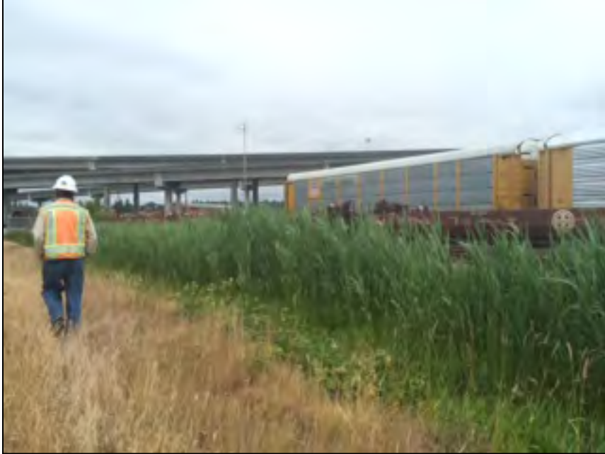
Photo 1. Tall grass growing in drainage ditch. Grass is maintained annually.
