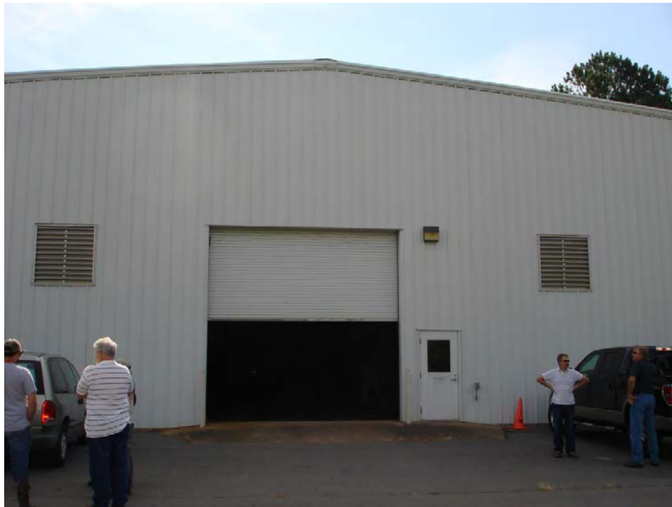
Photograph No. 2 Site: Vertac Inc. Superfund Site Description: Front entryway of the Wastewater Treatment Plant (WWTP) Date: June 4, 2013 Direction: East
