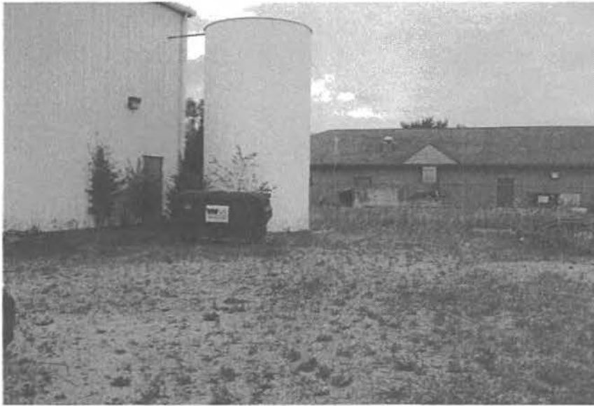
Picture 6 – General Site conditions within the fence
