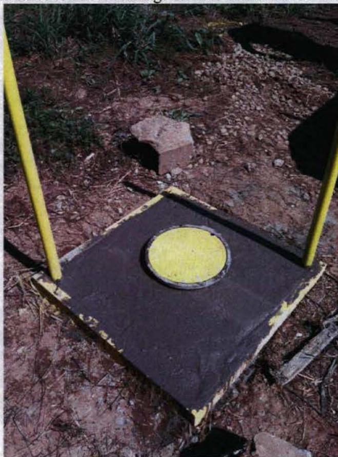
Monitoring well 2D being repaired.
