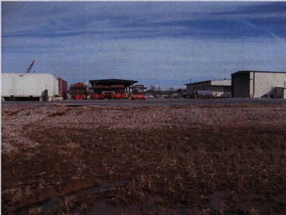
Looking across the Site from south to north.
