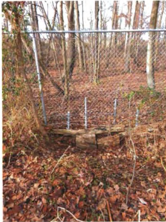
Fence repair at Landfill No. 2.
