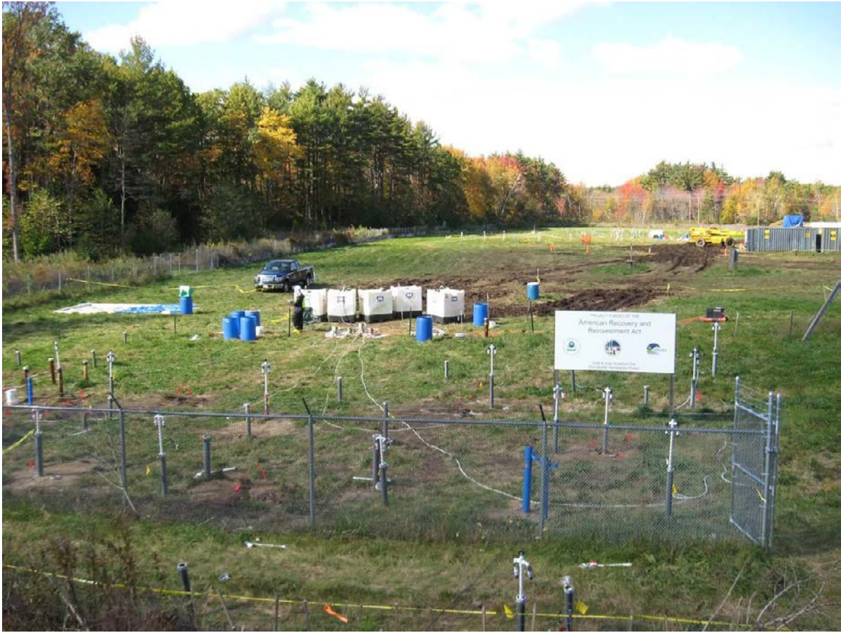
View from Route 125 During ISCO Injections, Fall 2009
