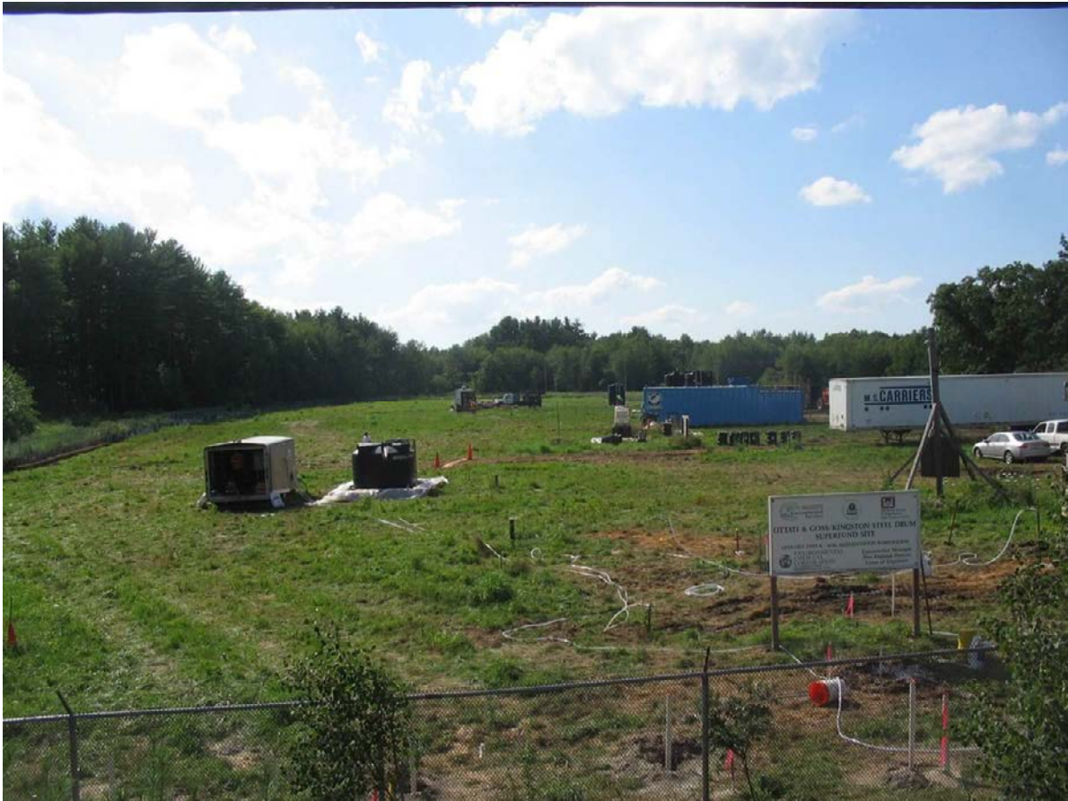
View from Route 125 During ISCO Injections, Fall 2008
