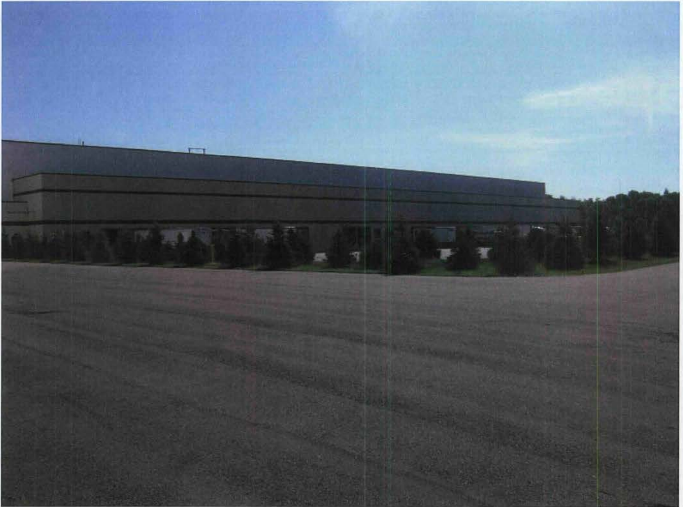
Chemtool as seen from Pump Building
