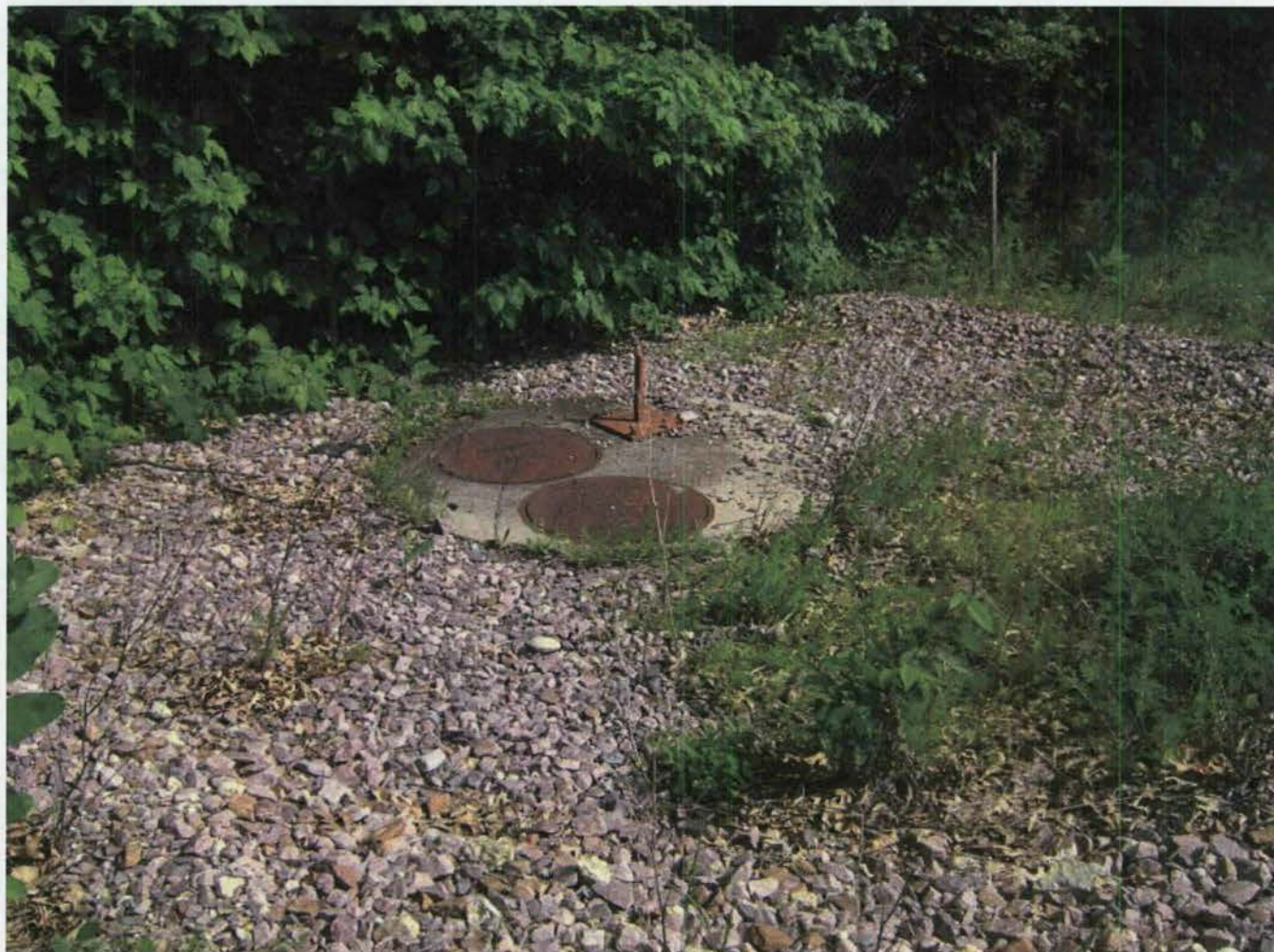
Effluent Manhole
