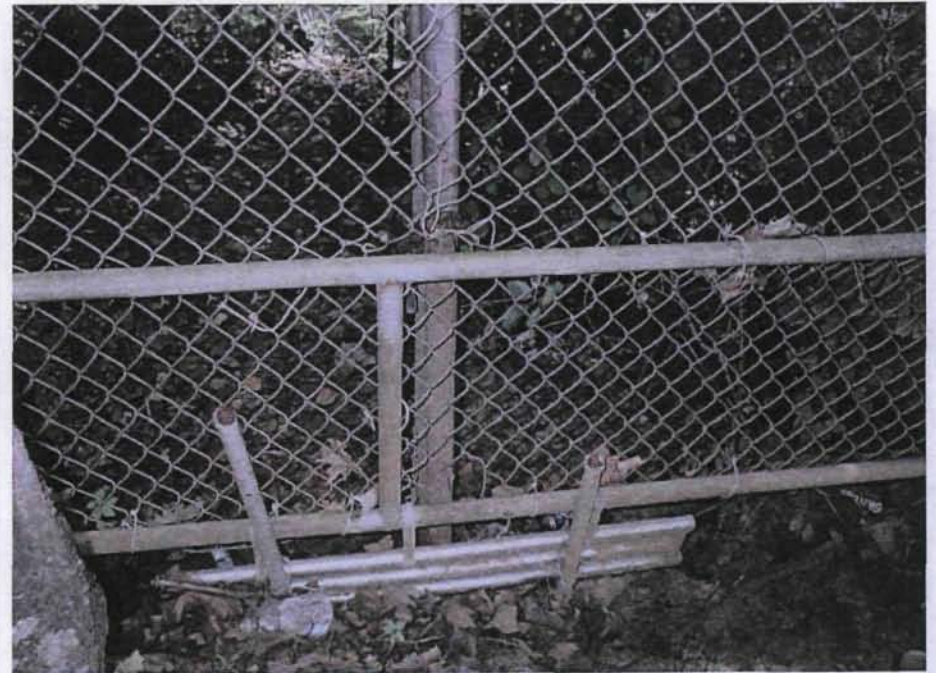
Photo 10: Area of fence line along the eastern perimeter where the city of Elyria was able to block access through the gap beneath fence line.
