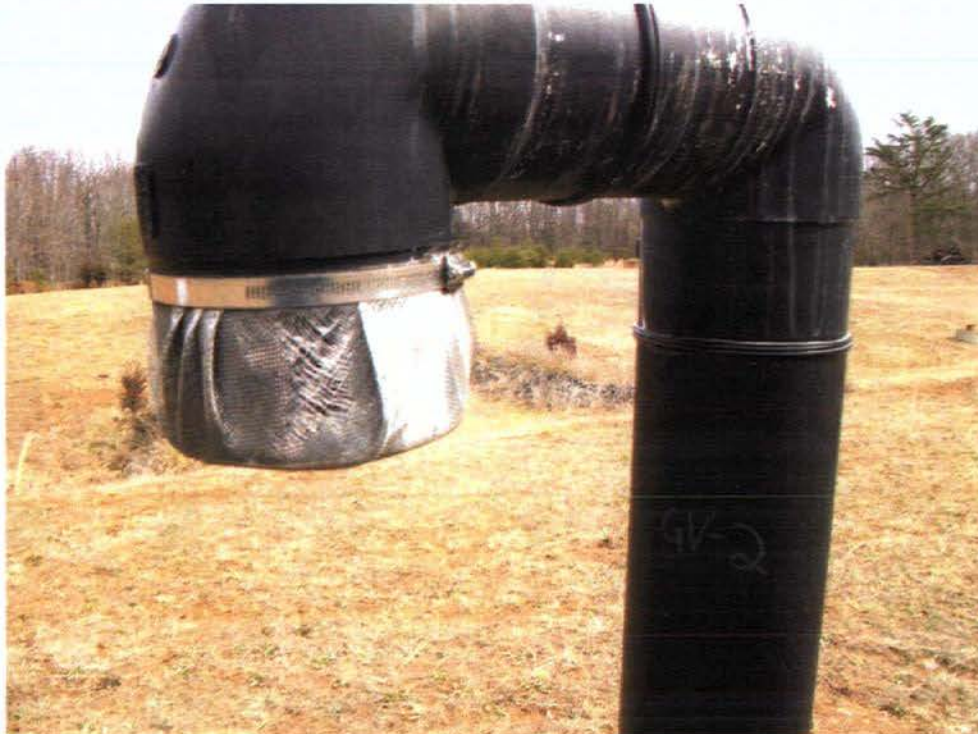
Photo: 196 Date: 02/28/13 Description: Facing north at Landfill. Gas vent, GV-2, with damage to vent screen. Over grown vegetation in drainage swale in background. Photographer: Rich Opem
