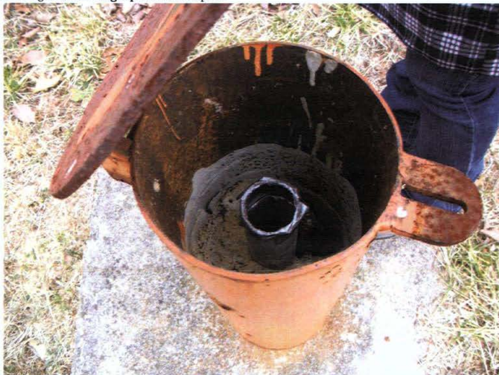
Photo: 232 Date: 02/28/13 Description: At monitoring well, MW-3B. Well pipe missing cap. Photographer: Rich Opem
