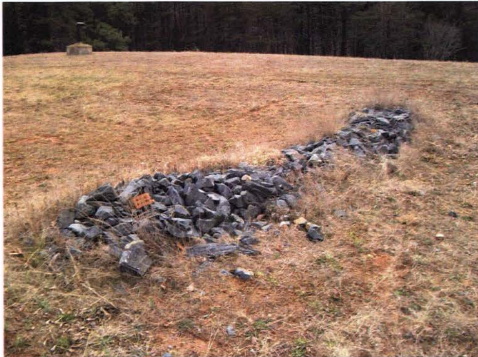
Photo: 202 Date: 02/28/13 Description: Near GV-2 at Landfill. Over grown vegetation within rock dam. Photographer: Rich Opem
