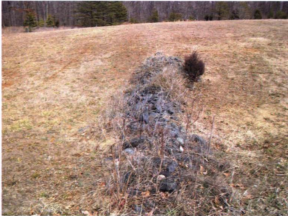
Photo: 199 Date: 02/28/13 Description: Near GV-2 at Landfill. Over grown vegetation within rock dam. Photographer: Rich Opem
