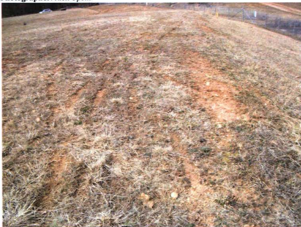
Photo: 213 Date: 02/28/13 Description: Facing northwest at Landfill near GV-6. Bare grass spots on Landfill cover in need of reseeding. Photographer: Rich Opem
