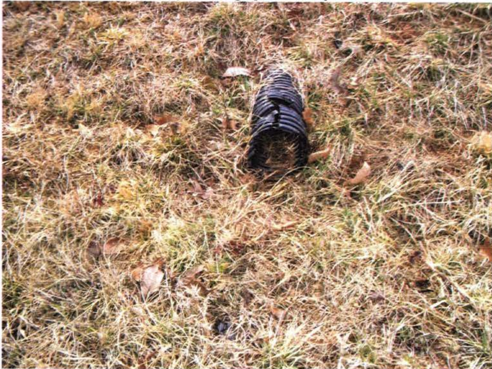
Photo: 211 Date: 02/28/13 Description: Facing northeast at landfill near GV-6. damaged drainage pipe. Photographer: Rich Opem
