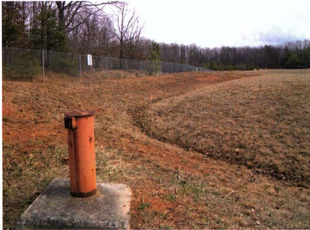
Photo: 189 Date: 02/28/13 Description: Facing northeast at Landfill near back gate fence. Monitoring well MW-3B. Well has no lock and well cap. Photographer: Rich Opem
