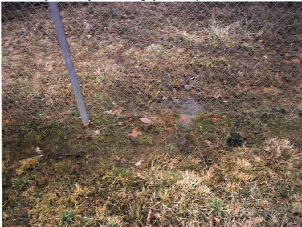
Photo: 225 Date: 02/28/13 Description: Southwest area of Landfill long south fence line. Standing water and gap at bottom of fence. Photographer: Rich Opem
