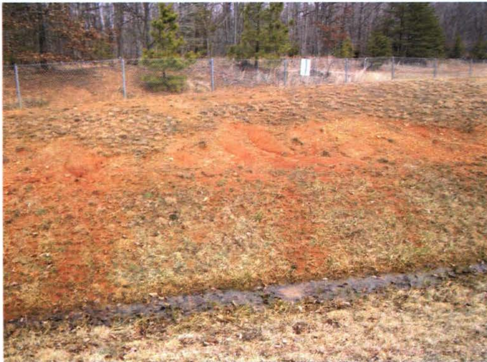
Photo: 194 Date: 02/28/13 Description: Facing north at Landfill near GV-1. Bare grass spots in need of reseeding and standing water. Photographer: Rich Opem
