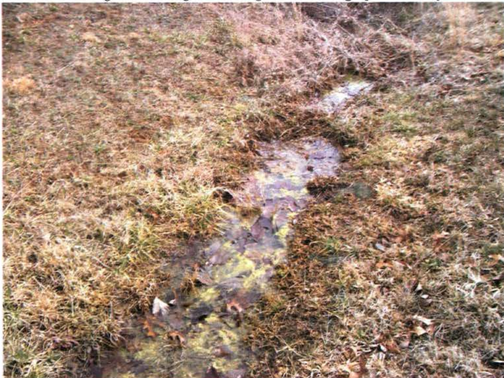
Photo: 198 Date: 02/28/13 Description: Near GV-2 at Landfill. Standing water and algae in drainage swale. Photographer: Rich Opem
