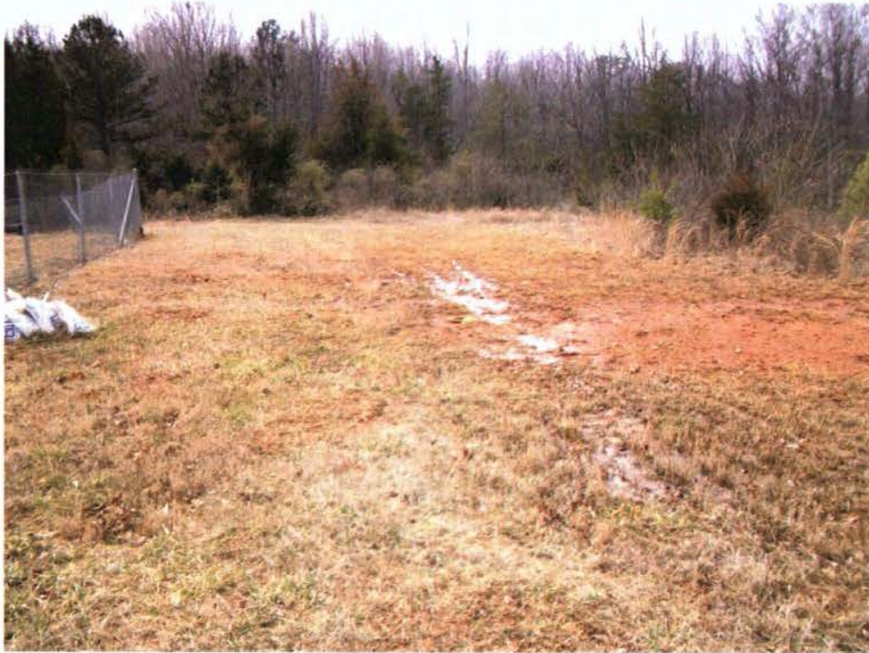
Photo: 184 Date: 02/28/13 Description: Facing southwest near back Landfill gate and beyond fence. Left over bags of sand; bare grass spots in need of reseeding; low spot with standing water. Photographer: Rich Opem
