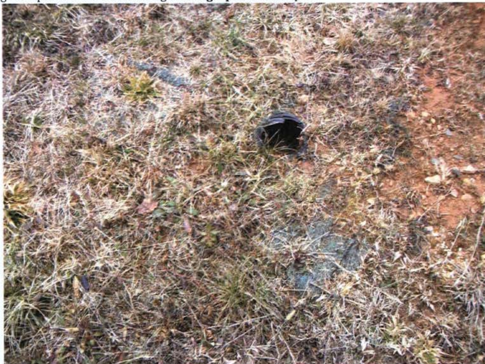
Photo: 230 Date: 02/28/13 Description: Inverted drainage pipe near bare grass spot in need of reseeded. Located at southeast corner of Landfill. Photographer: Rich Opem
