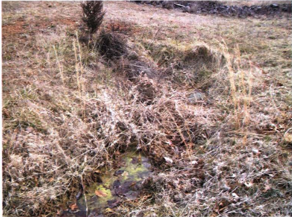
Photo: 197 Date: 02/28/13 Description: Over grown vegetation in drainage swale and rock dam near GV-2. Standing water and algae in drainage swale. Photographer: Rich Opem
