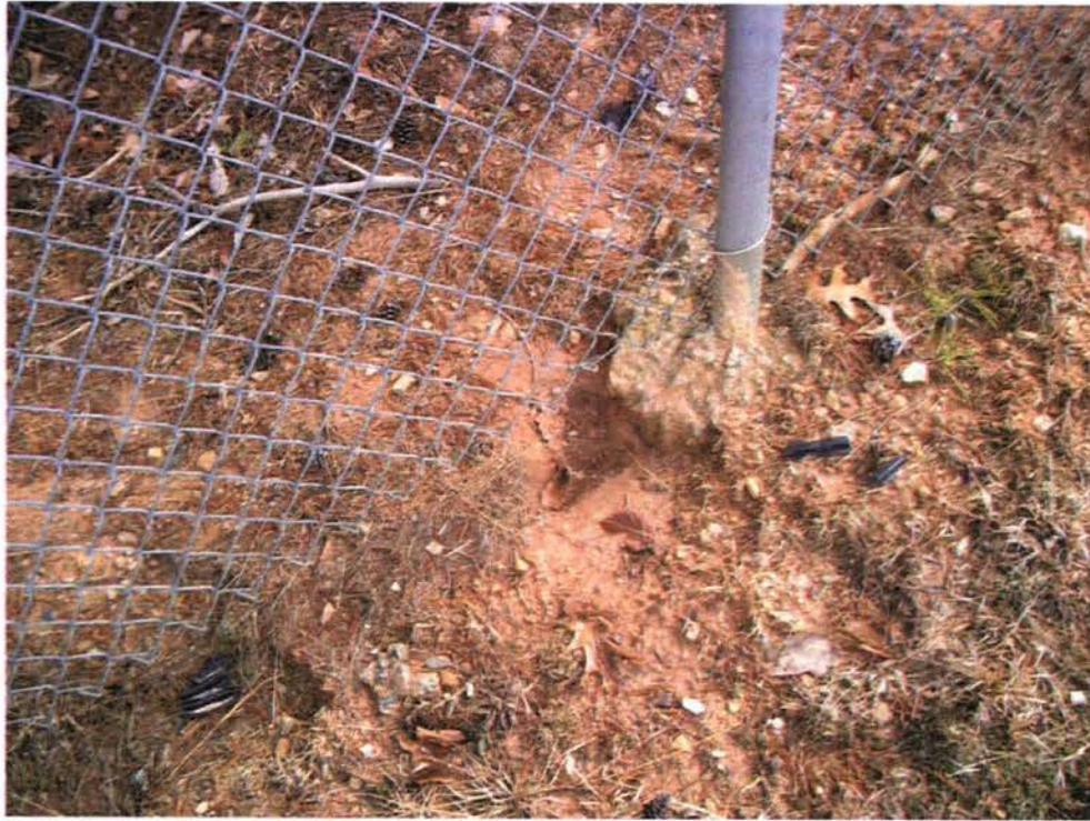
Photo: 210 Date: 02/28/13 Description: Facing northeast at Landfill fence near GV-6. Gap at bottom of fence and bare grass spot. Photographer: Rich Opem
