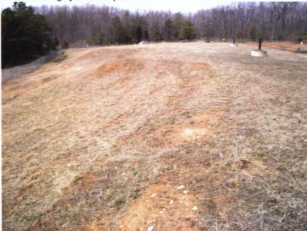
Photo: 203 Date: 02/28/13 Description: Facing west at Landfill near south of Landfill fence line. Several bare grass spots on landfill cover in need of reseeding. Standing water near southwest corner of fence line. Photographer: Rich Opem
