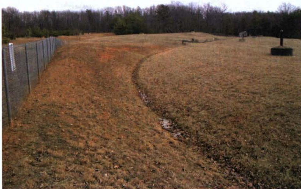
Photo: 190 Date: 02/28/13 Description: Facing east at Landfill. Landfill with bare grass spots near north fence line. Standing water, drainage swale and gas vents (GV-1 and GV-2) in the background. Photographer: Rich Opem
