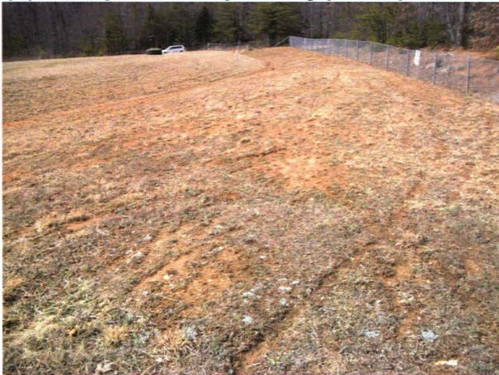
Photo: 220 Date: 02/28/13 Description: Facing west at Landfill near northeast fence line. Bare grass spots in need of reseeding. Photographer: Rich Opem
