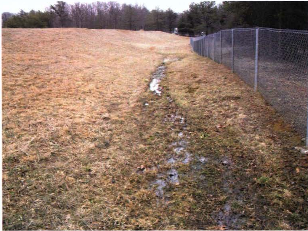
Photo: 224 Date: 02/28/13 Description: Facing east of Landfill near south fence line. Standing water with algae in drainage swale. Photographer: Rich Opem
