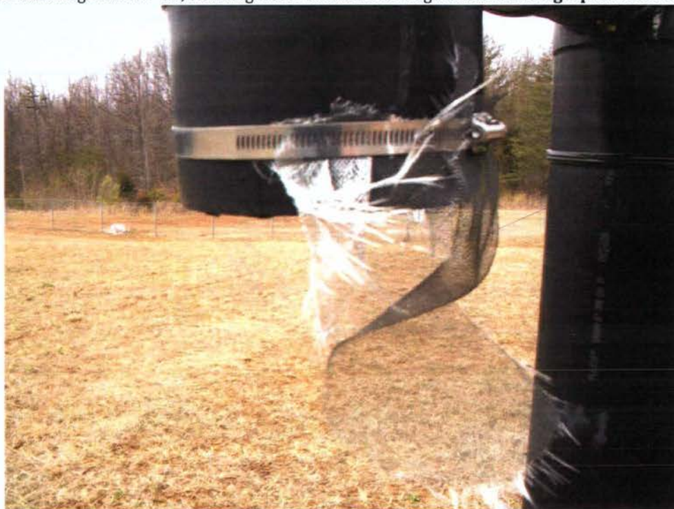
Photo: 192 Date: 02/28/13 Description: Facing northwest at Landfill. Damaged vent screen at gas vent, GV-1. Photographer: Rich Opem
