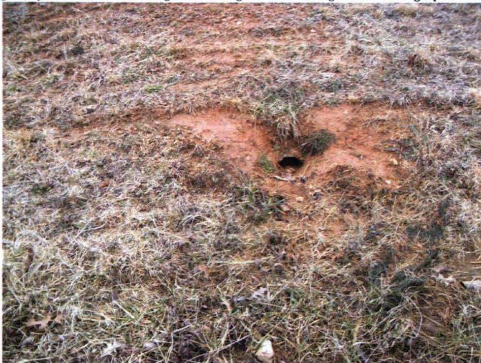
Photo: 223 Date: 02/28/13 Description: Bare grass spot around clogged drainage pipe. Located at northwest corner of Landfill. Photographer: Rich Opem
