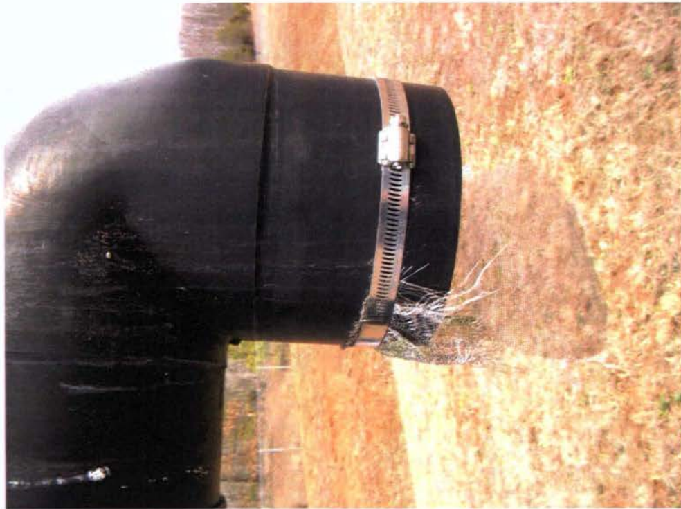
Photo: 193 Date: 02/28/13 Description: Damaged vent screen at gas vent, GV-1. Photographer: Rich Opem
