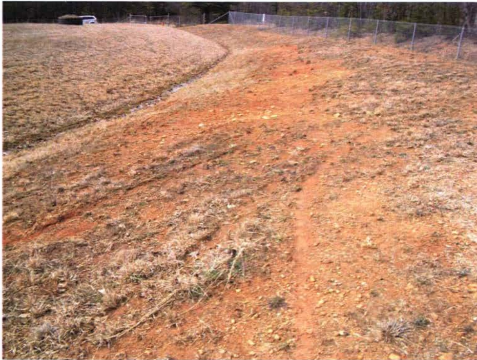
Photo: 221 Date: 02/28/13 Description: Facing northwest at Landfill near north fence line. Bare grass spots in need of reseeding and standing water in drainage swale. Photographer: Rich Opem
