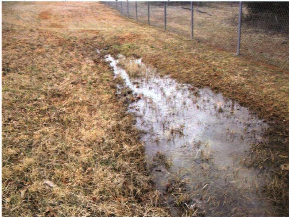
Photo: 227 Date: 02/28/13 Description: Facing southeast of Landfill near south fence line. Standing water in drainage swale. Photographer: Rich Opem
