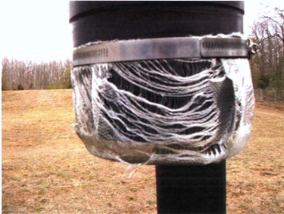
Photo: 205 Date: 02/28/13 Description: On Landfill. Gas vent, GV-4, with damaged vent screen. Photographer: Rich Opem
