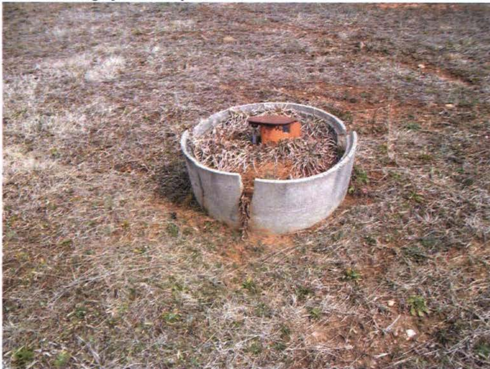
Photo: 200 Date: 02/28/13 Description: On Landfill. Monitoring well, MW-2SU, damaged protective concrete ring around well. Photographer: Rich Opem
