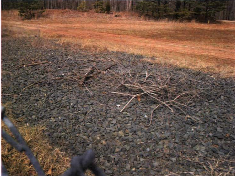
Photo: 216 Date: 02/28/13 Description: Facing north near fence line. Riprap area in good condition with shrub growth. Photographer: Rich Opem
