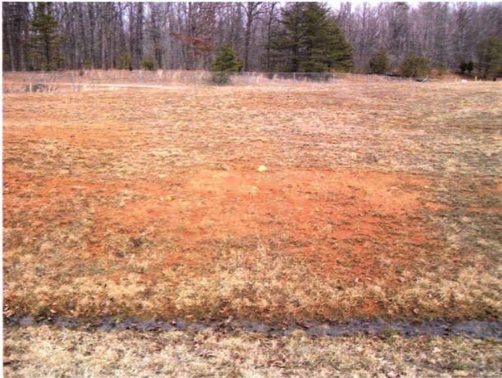
Photo: 195 Date: 02/28/13 Description: Facing north at Landfill. Bare grass spots in need of reseeding. Standing water. Photographer: Rich Opem
