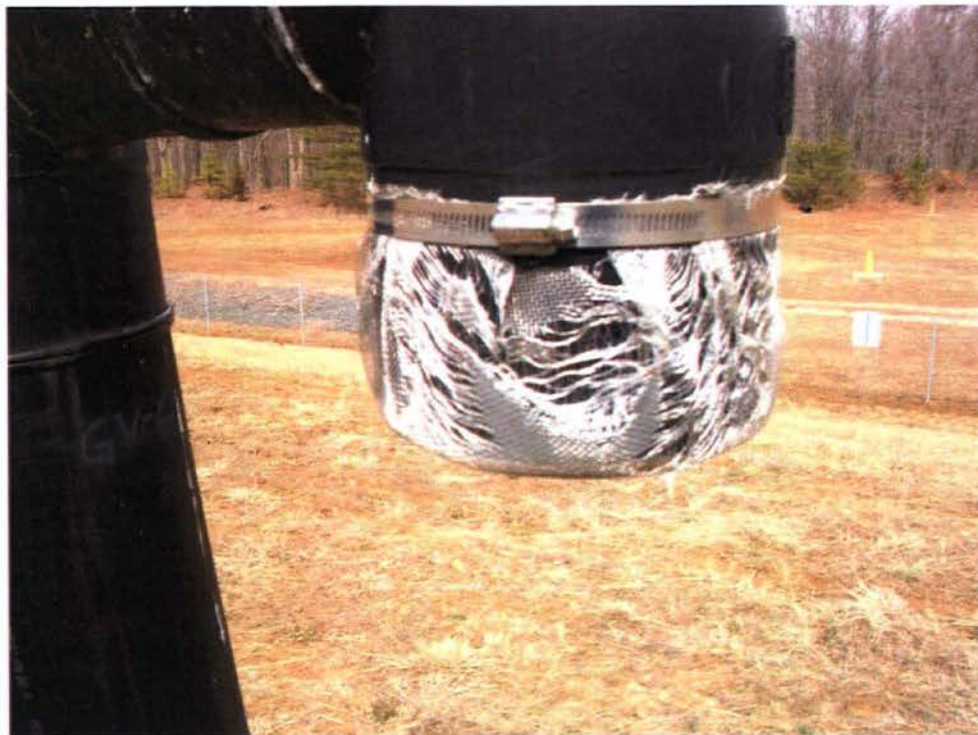
Photo: 212 Date: 02/28/13 Description: On Landfill. Gas vent, GV-6, with damaged vent screen. Photographer: Rich Opem
