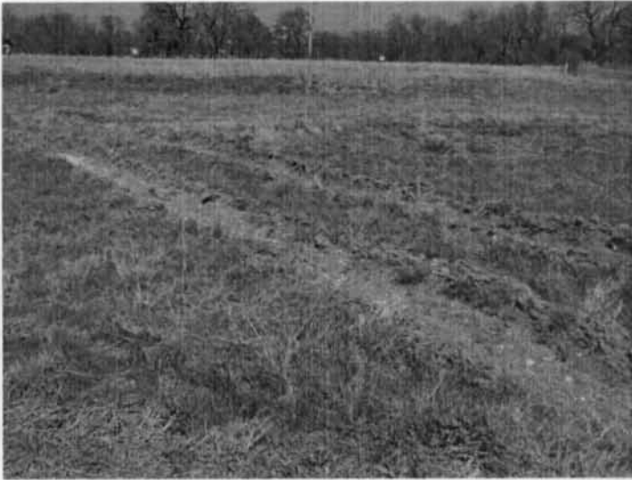
Photo 47. Wheel ruts and grass cover damage in the area between the paved parking area and the EVL in the background.
