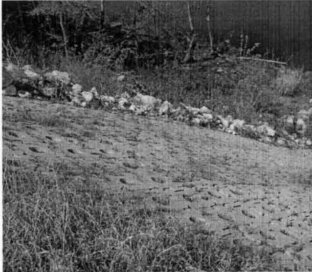
Photo 35. Western edge of the stabilized Leon River bank.
