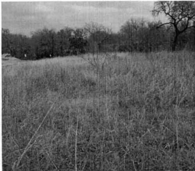
Photo 53. Grass cover on the top of the CSP.
