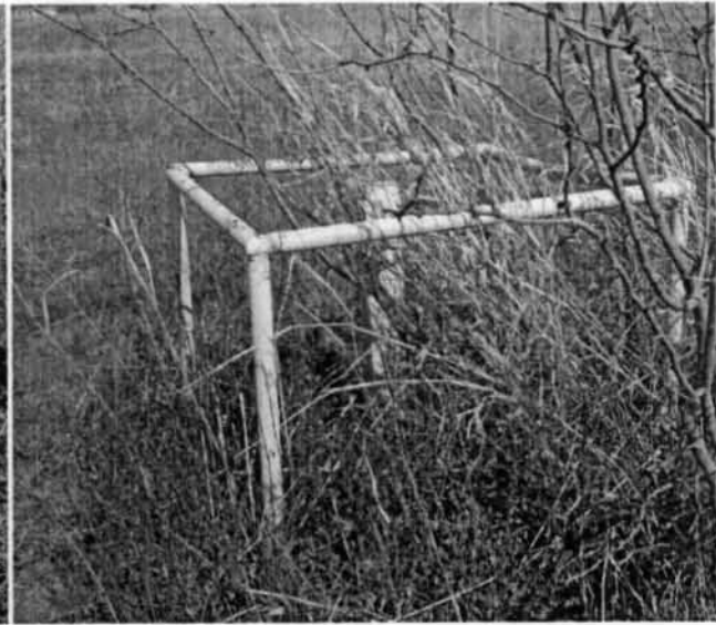
Photo 8. MW-17, has no identification marker, overgrown
