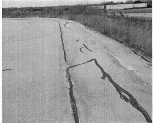
Photo 59. Patched cracks and asphalt repair area.
