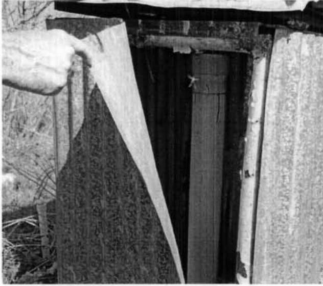
Photo 1. MW-07, no identification marker, enclosed in a corrugated metal housing.
