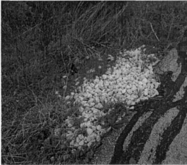
Photo 62. Rip rap along the southern edge of the CC.
