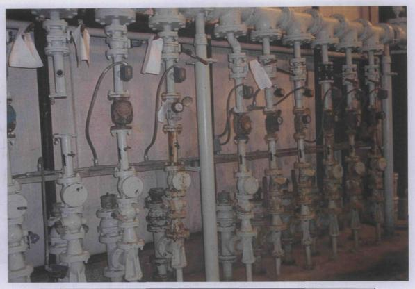
Photo ID Description: Groundwater flow meters inside treatment building
