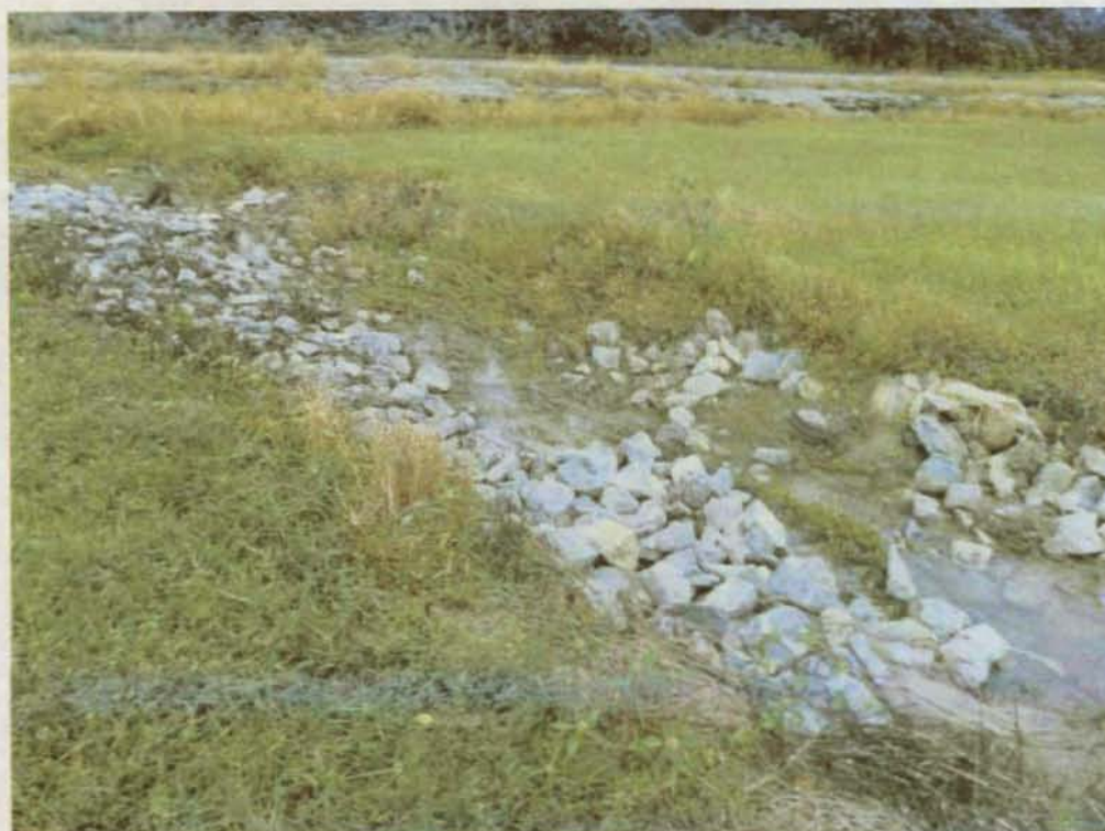
Ditch along OUI where soil removal was conducted.
