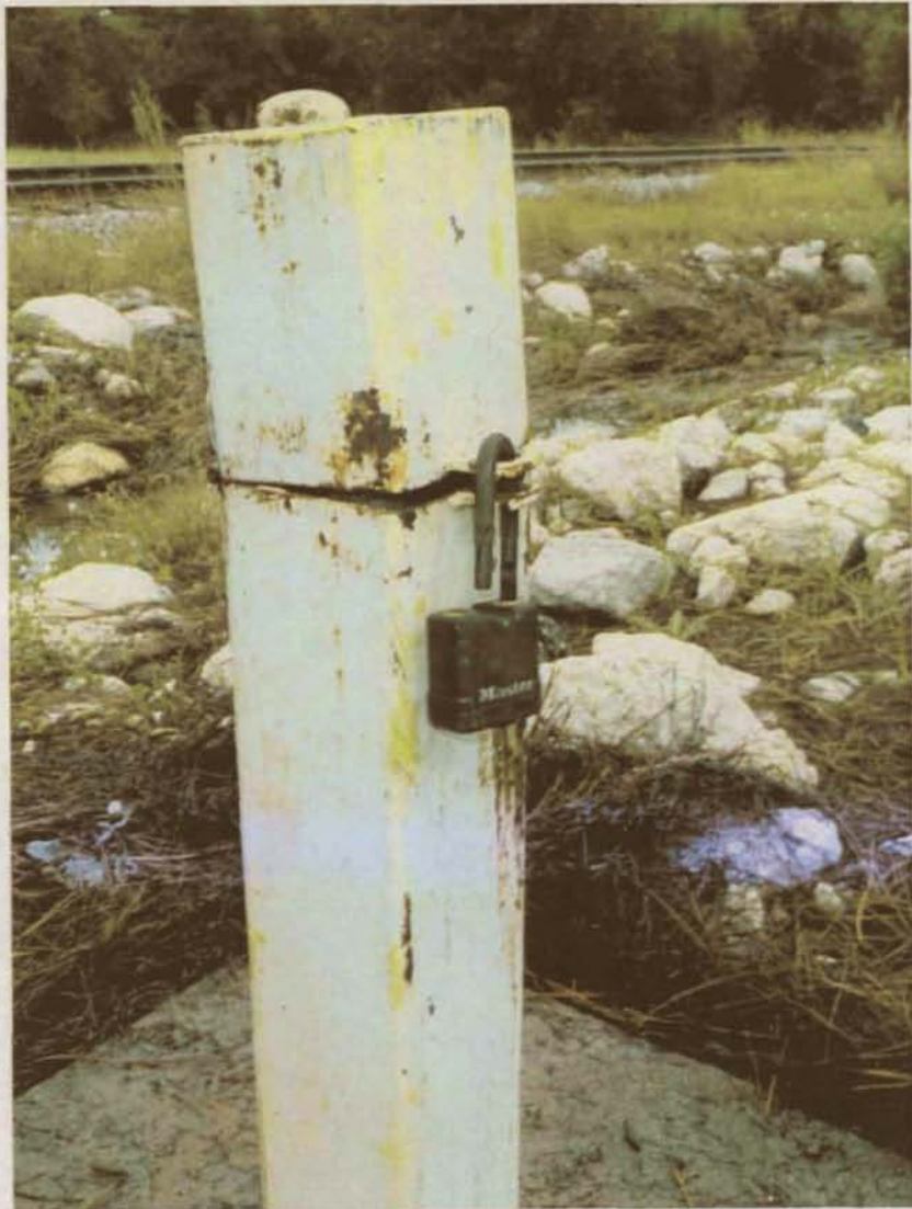
Unlabeled, unlocked monitoring well for MNA at OU2.
