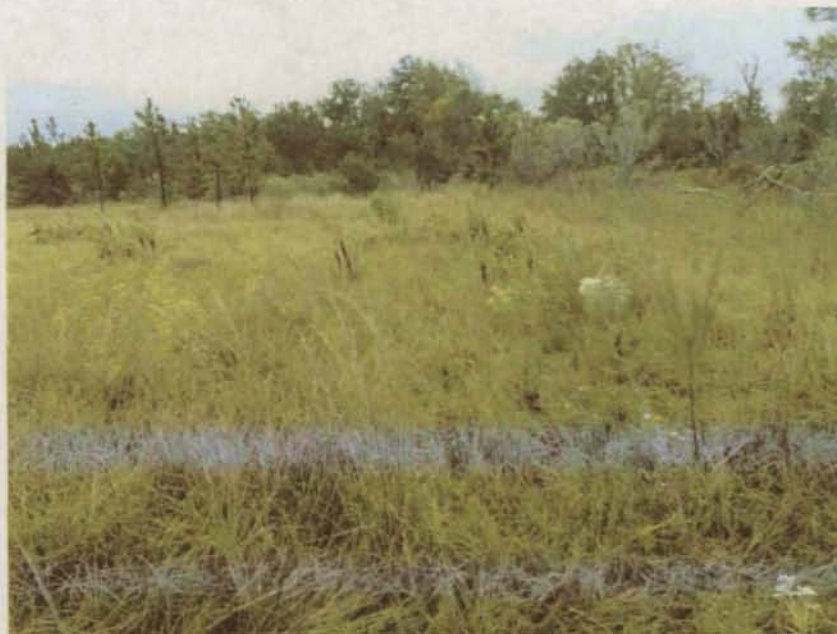
Underground barrier and trench for collection of ground water in the F&G system.
