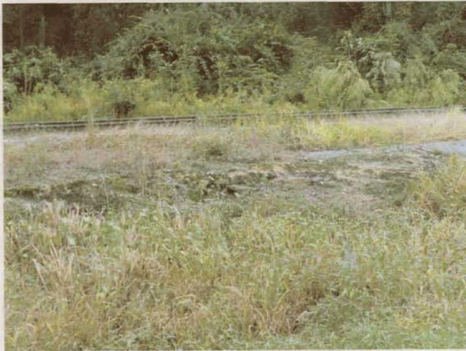
Ditch and erosion along railroad tracks.
