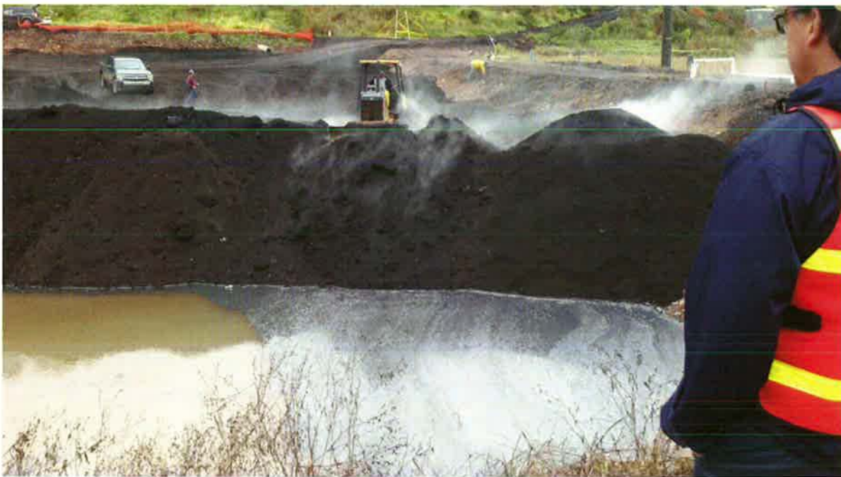
OU#4 – East Cinderbank Remedial Interim Measure cell IRM backfilling cont.
