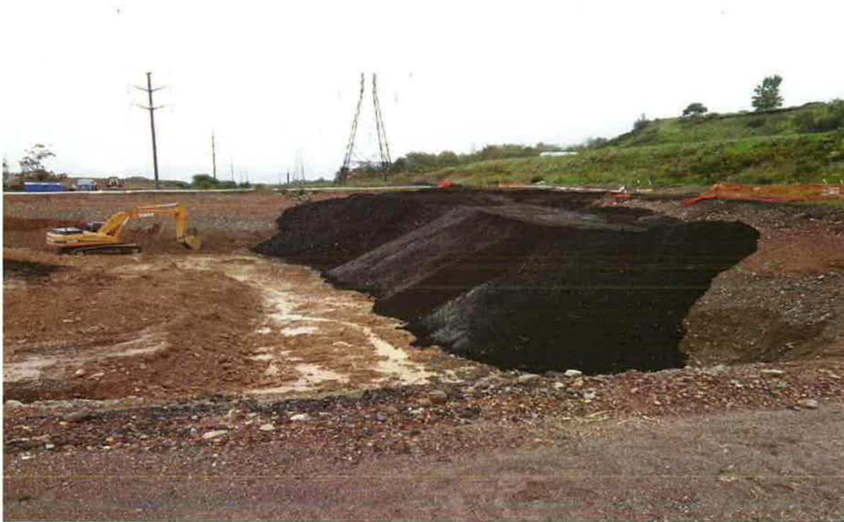
OU#4 – East Cinderbank Remedial Interim Measure cell IRM backfilling
