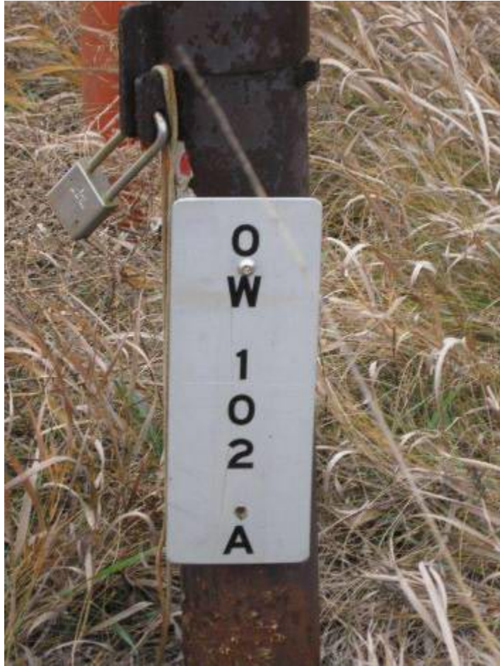
Groundwater monitoring well
