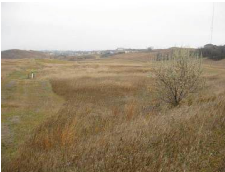
Landfill and monitoring well
