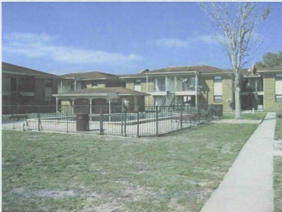
Swimming pool courtyard
