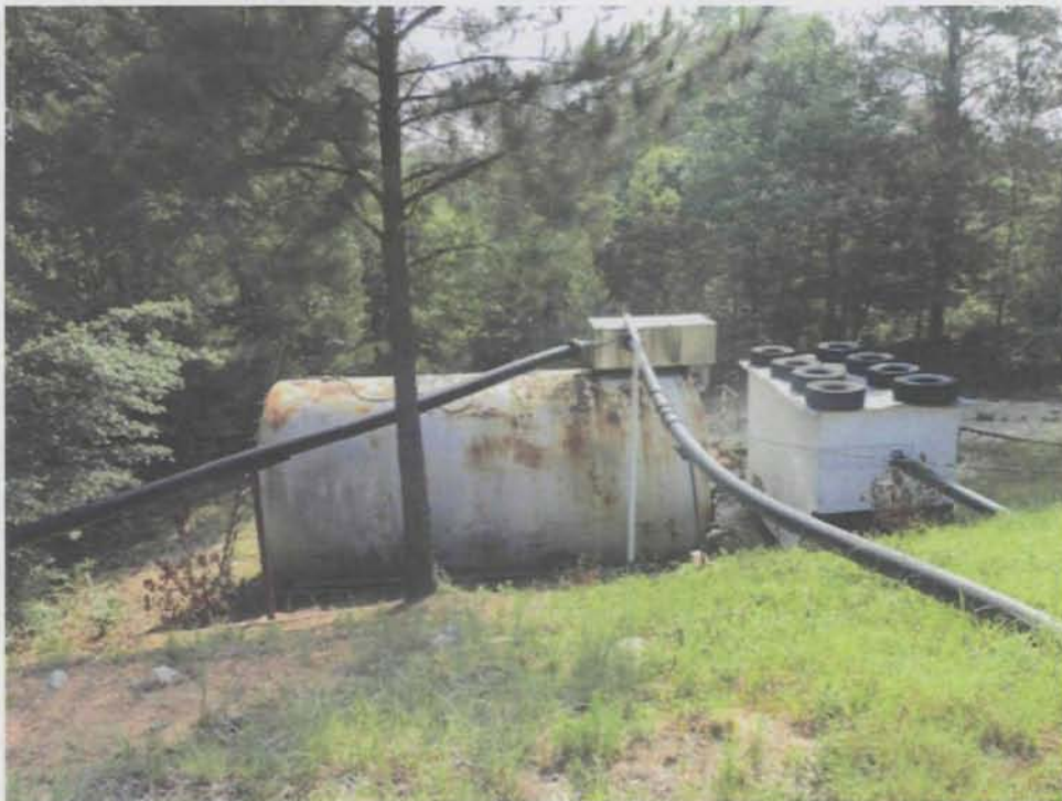
Backup transfer system (12,000-gallon tank and two pumps)
