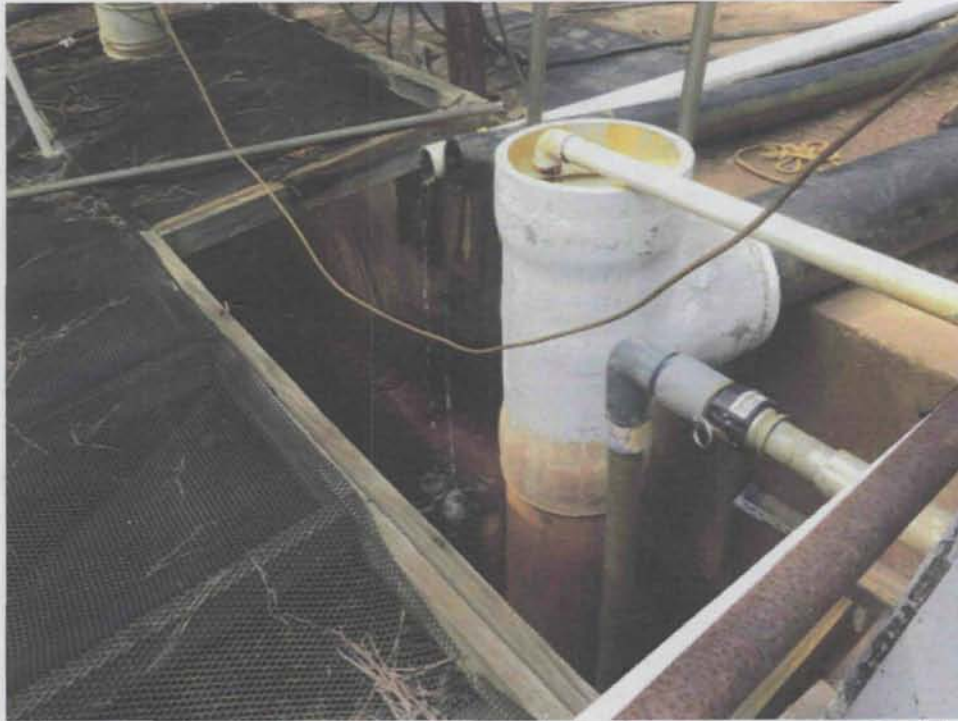
Pad 6 pump where seepage from pad 6 pond dam and below the dam is captured and pumped back into the pad 6 pond
