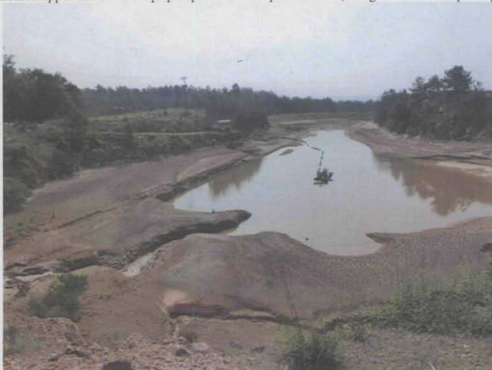
Northwest Trend pit (settling site for neutralization treatment sludge)
