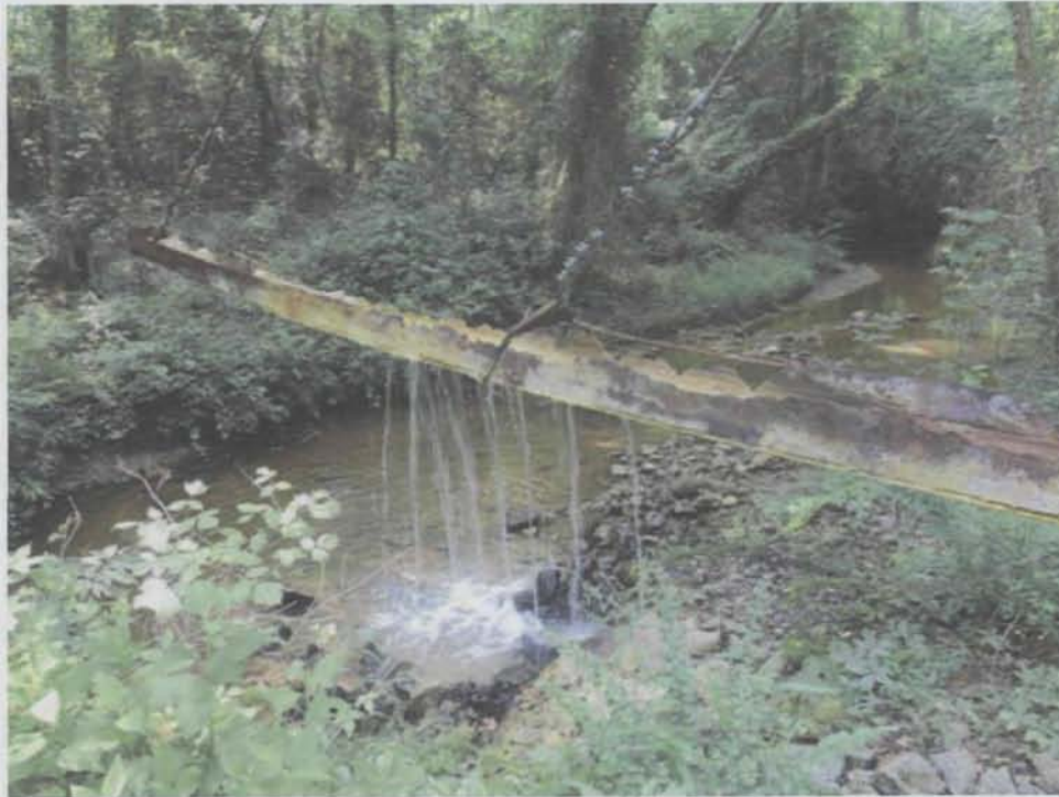
Treated effluent discharge to Little Fork Creek
