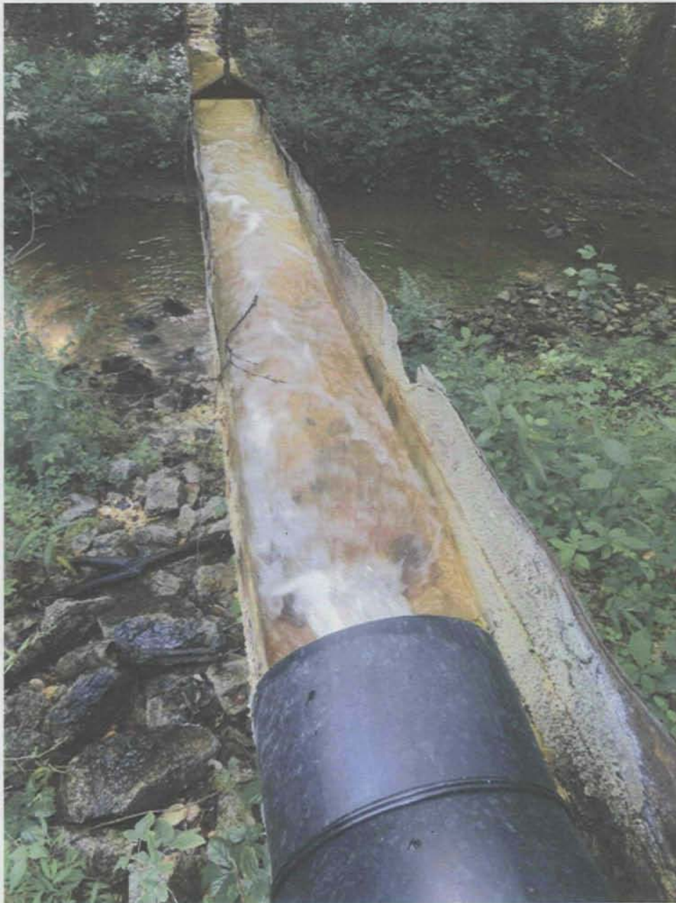
Treated effluent discharge to Little Fork Creek
