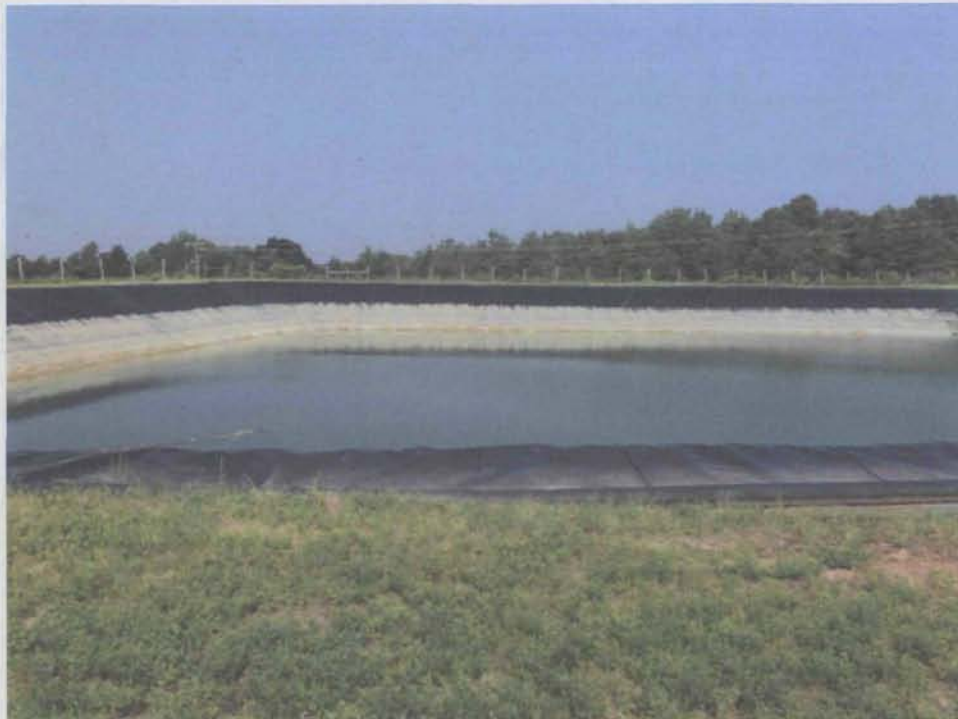
Treated water holding pond (plastic liner used to store discharge-quality water)
