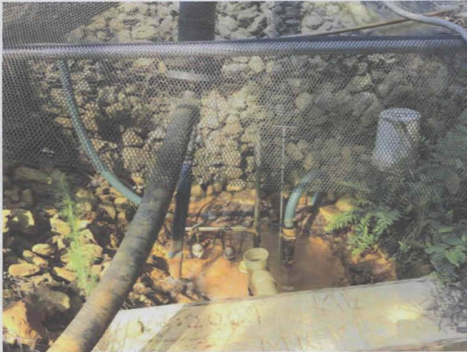
Combined upper and lower seeps pump transfers seep water to 12,000 gallon tank and pad 6 pond
