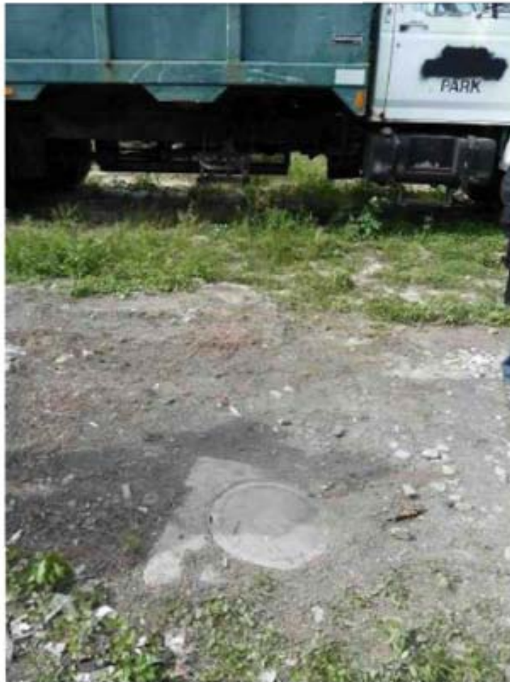
Monitoring wells cluster #1 on the Branif Auto Parts property.
