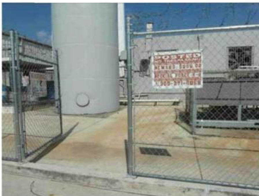
Warning sign and "no trespassing" sign.
