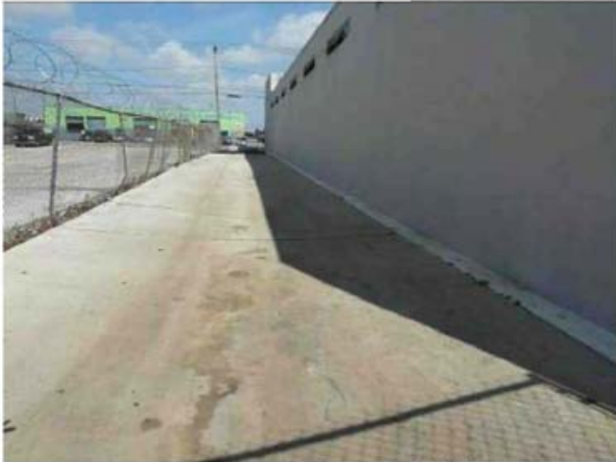
Cap on the west side of the Airco building.
