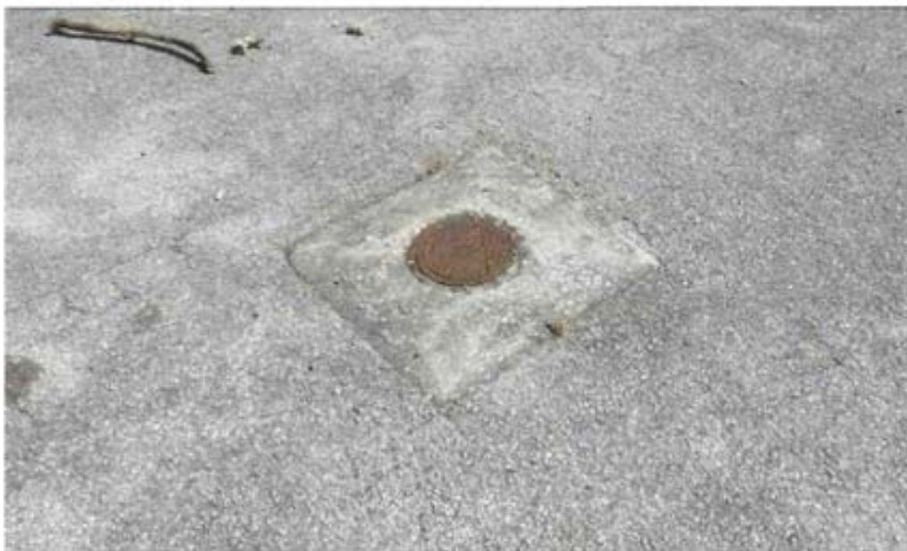
Unmapped monitoring well at neighboring parking lot.
