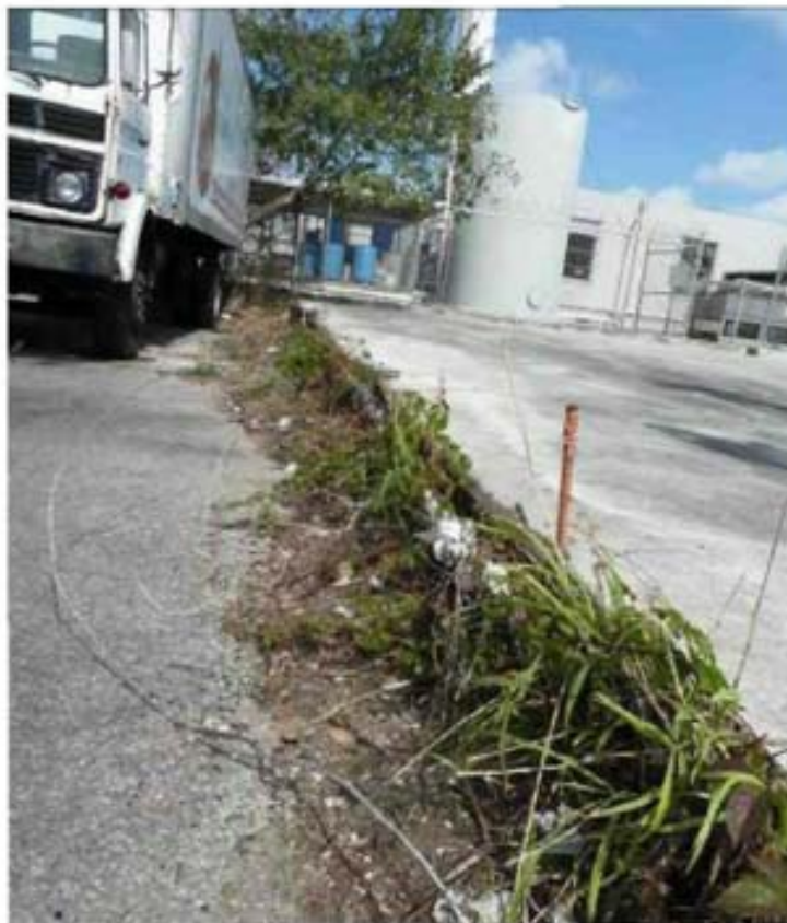
Cap on adjacent property where fence was removed.
