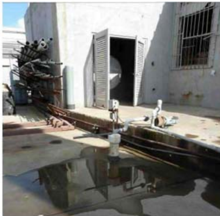
Recovery well (RW-4) within the Airco Plating Facility.
