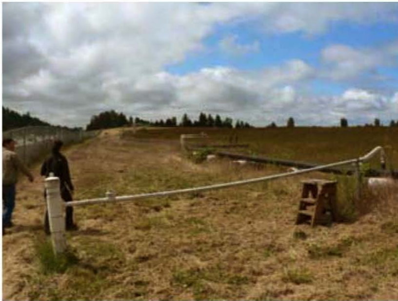
Landfill cover with gas extraction system.
