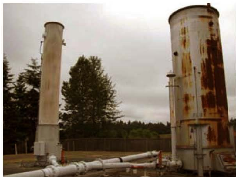
Gas extraction system flares. Current flare on left, backup flare on right.
