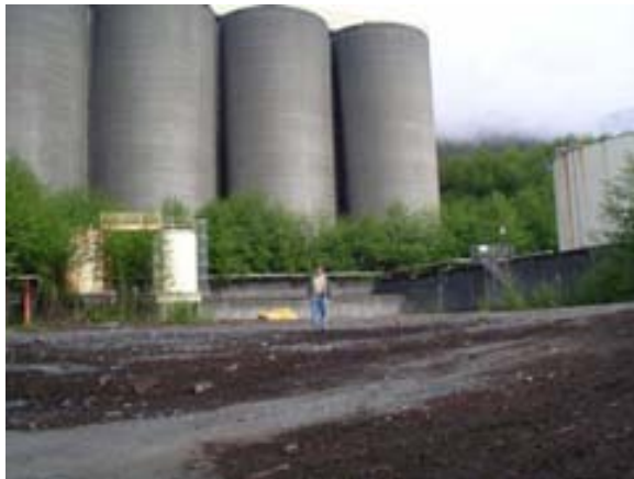
Photo 13. View north of silos
