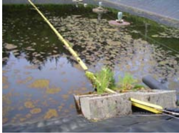
Photo 50. Aerators that were deactivated in 2007
