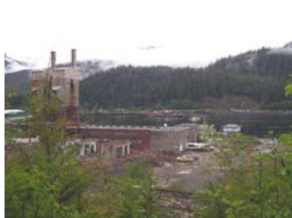
Photo 4. View southeast of demolished buildings from Administration building
