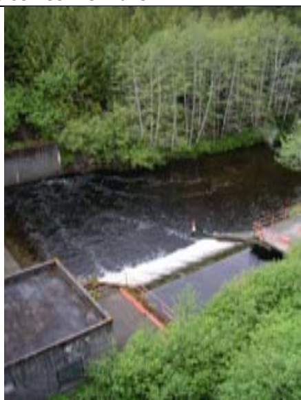
Photo 65. Outflow from dam into wood stave pipeline
