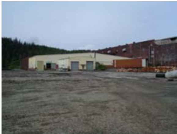
Photo 23. Leased warehouse on the northeast section of the Uplands Unit
