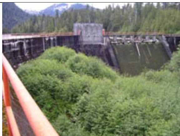
Photo 62. Connell Lake Dam
