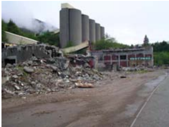
Photo 11. View northeast of demolished buildings and silos
