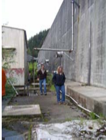
Photo 32. Outside wall of the wastewater treatment area
