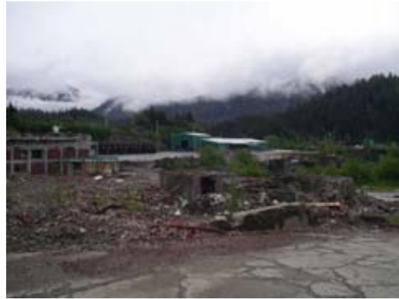
Photo 8. View east of demolished buildings
