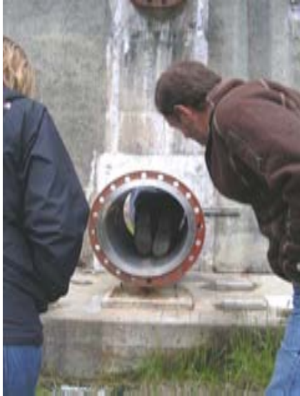
Photo 31. Climbing into the clarifier of the wastewater treatment area
