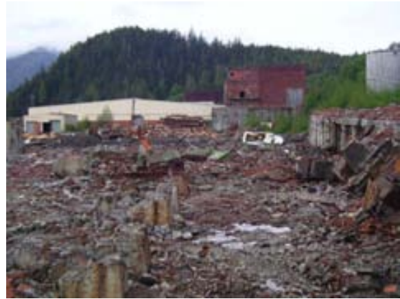
Photo 10. View west of demolished building where scrap metal has been removed for sale
