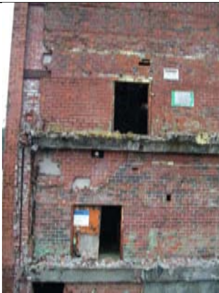
Photo 41. Outside wall of custom woodworking leased building
