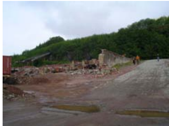
Photo 12. View northwest of demolished buildings
