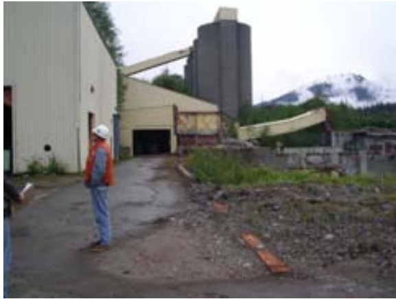
Photo 7. View east of silos
