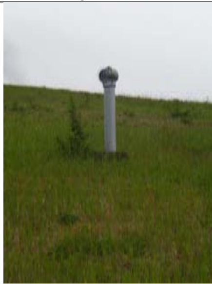
Photo 58. Close-up of landfill vent
