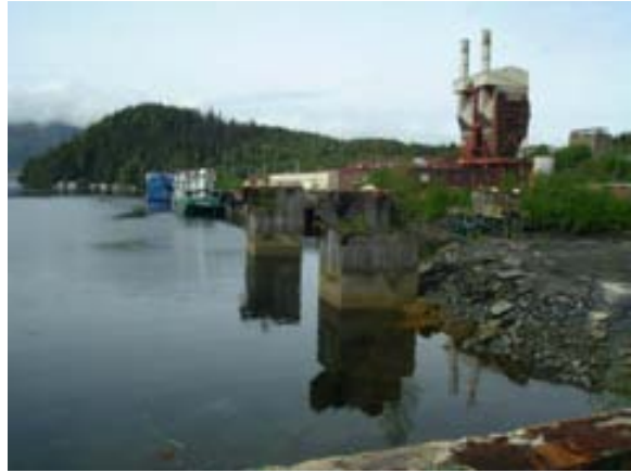
Photo 20. Remaining dock pilings for Ketchikan Pulp Mill
