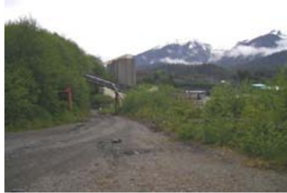
Photo 2. View east from Administration building downslope towards demolished buildings
