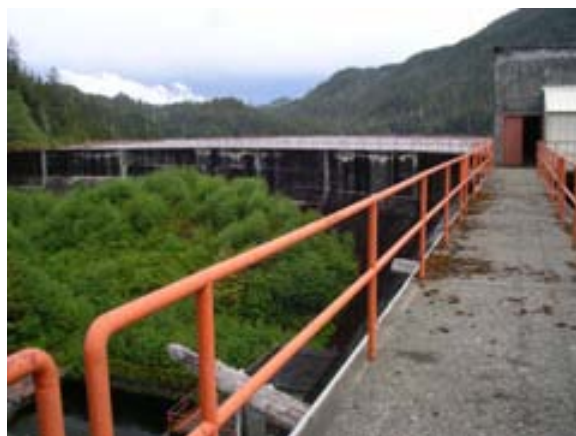
Photo 64. Walkway on the Connell Lake Dam
