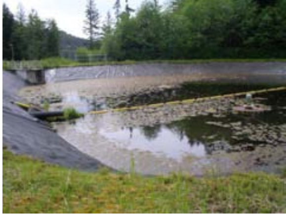
Photo. 49. Geomembrane lined sediment lagoon at the KPS landfill
