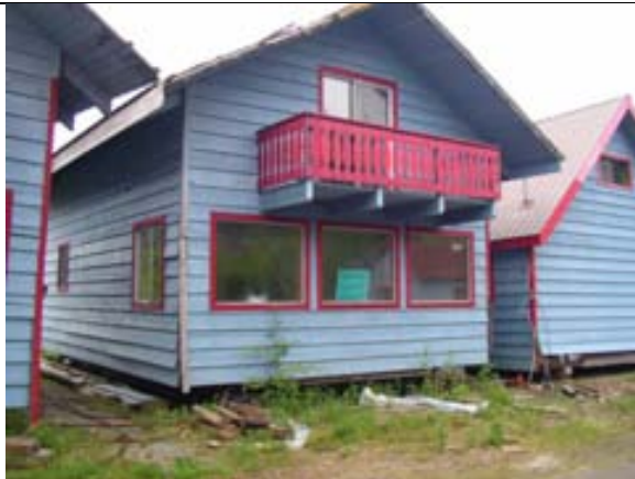
Photo 33. Leased Lighthouse Excursion building
