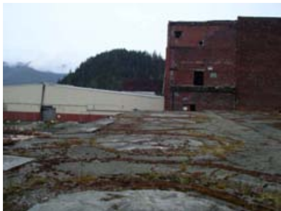
Photo 47. Panoramic view of the site facing west
