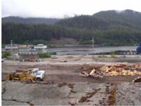
Photo 45. Panoramic view of the site facing south
