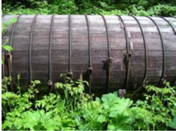
Photo 67. Close up of wood stave pipeline
