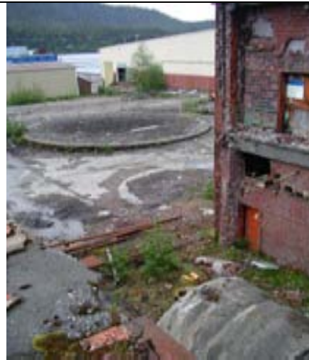
Photo 40. Roof of unused building
