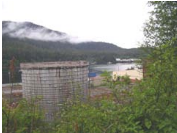
Photo 3. View southwest wood of stave tank from Administration building
