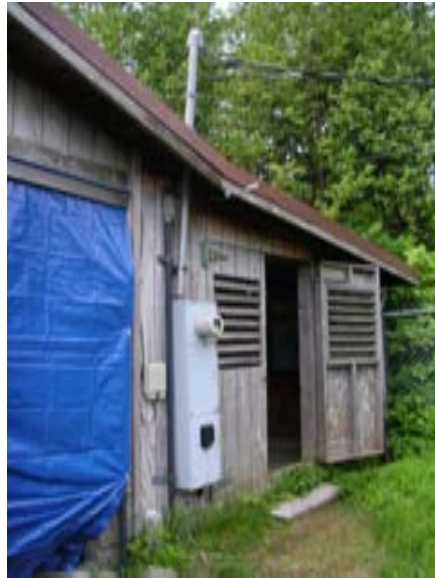
Photo 52. Landfill generator building
