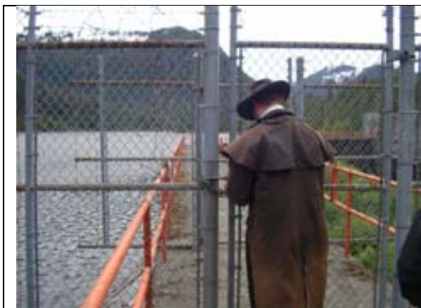
Photo 61. Gated and locked entry to the dam at Connell Lake.
