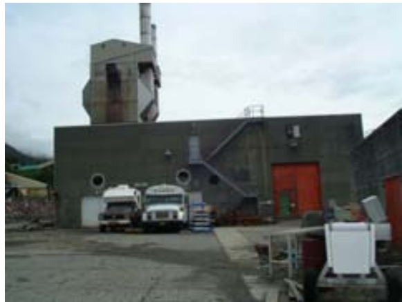
Photo 24. View east of building and electrostatic precipitators
