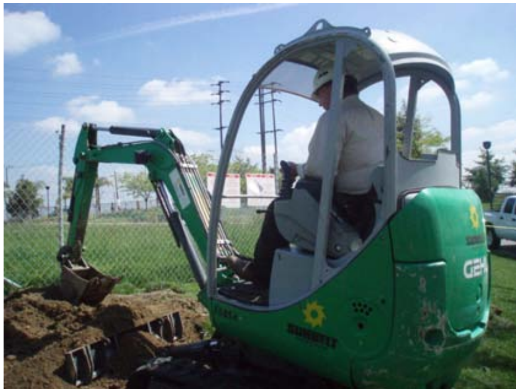
Photo 14: Jeff Waggle repairing well box at PB-04. May 26, 2010.
