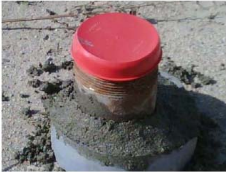
Caps and grout on electrode pipe taken March 10, 2010
