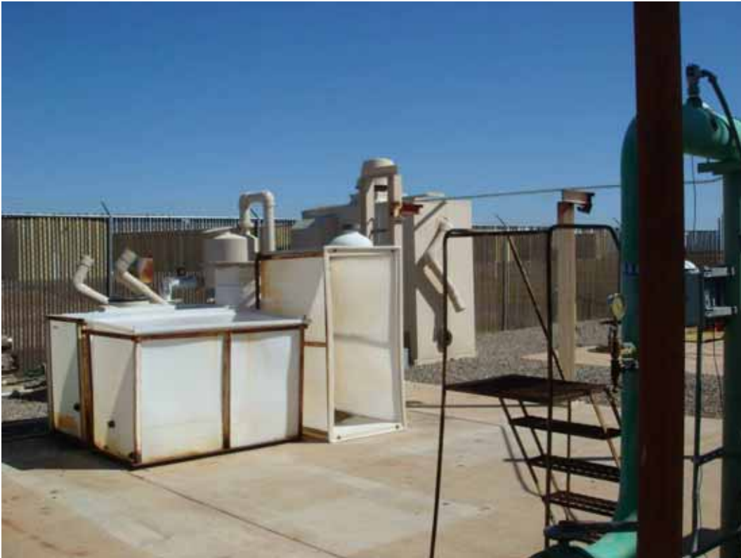
Photo 11. PGAS Site Visit. Subunit A treatment compound showing decommissioned equipment.
