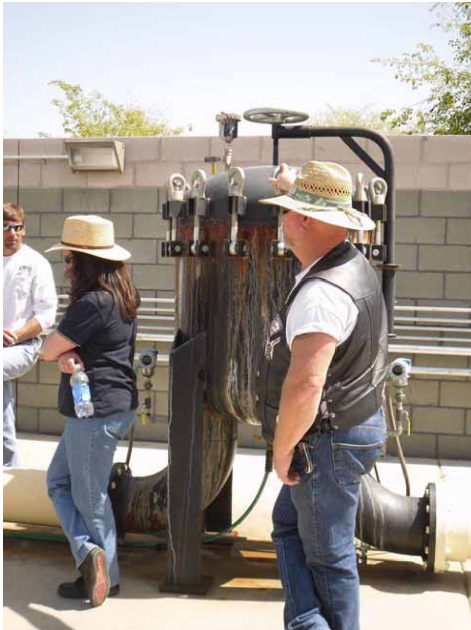
Photo 9. PGAN Site Visit. EA-06 influent bag filter housing (black vessel).
