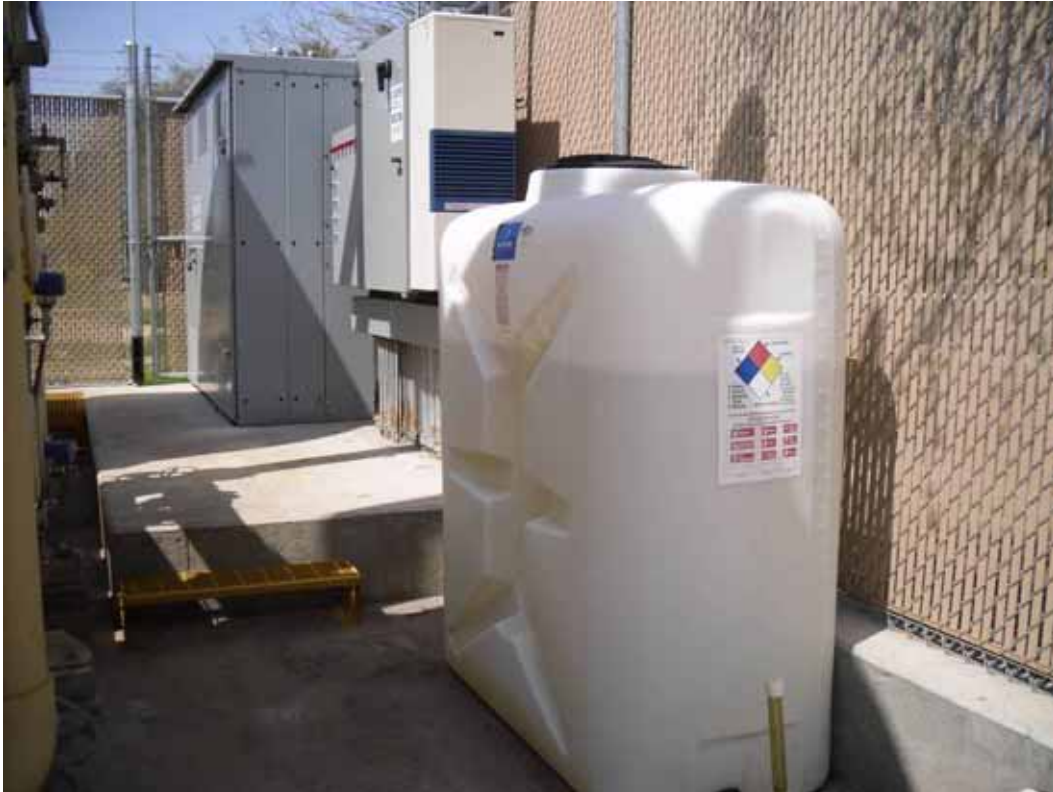
Photo 3. PGAN Site Visit. Sequestering agent, control panel, and motor control panel at EA-05.
