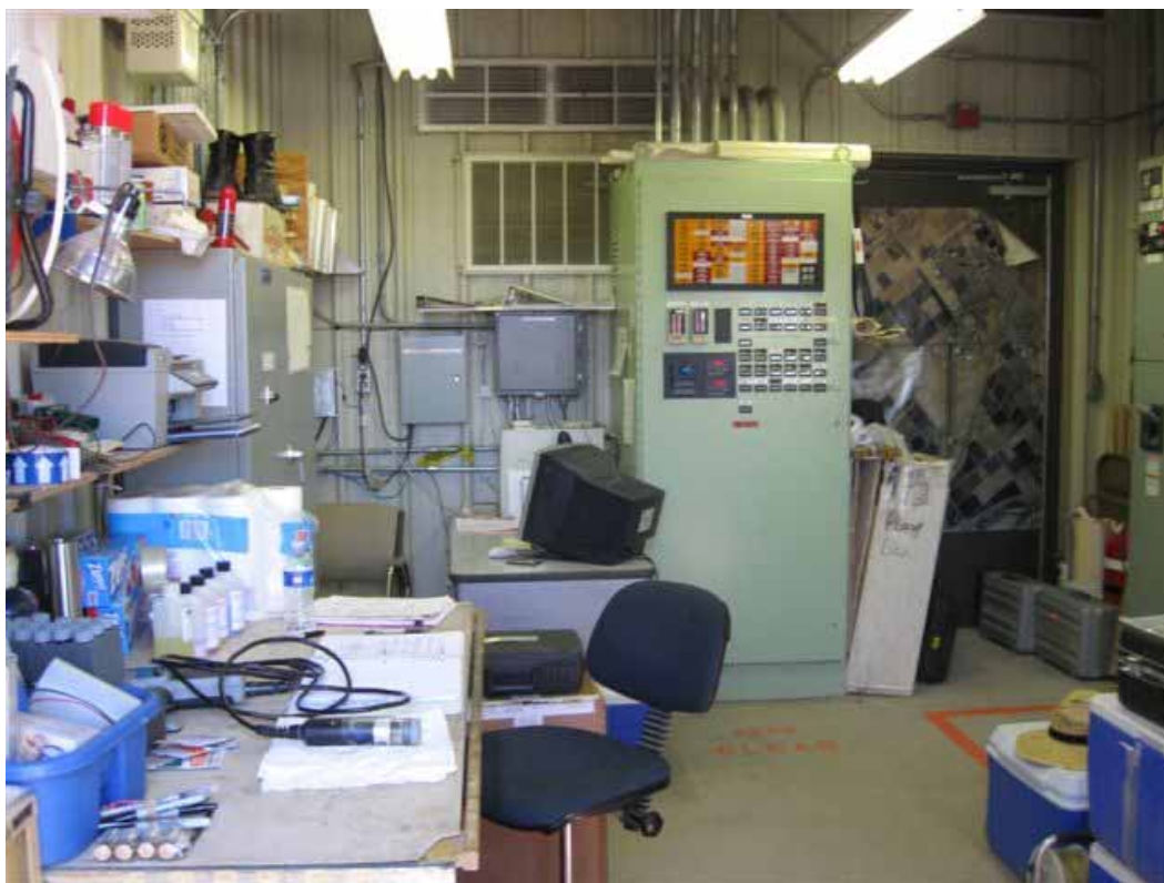
Photo 23. PGAS Site Visit. Subunit A control room.
