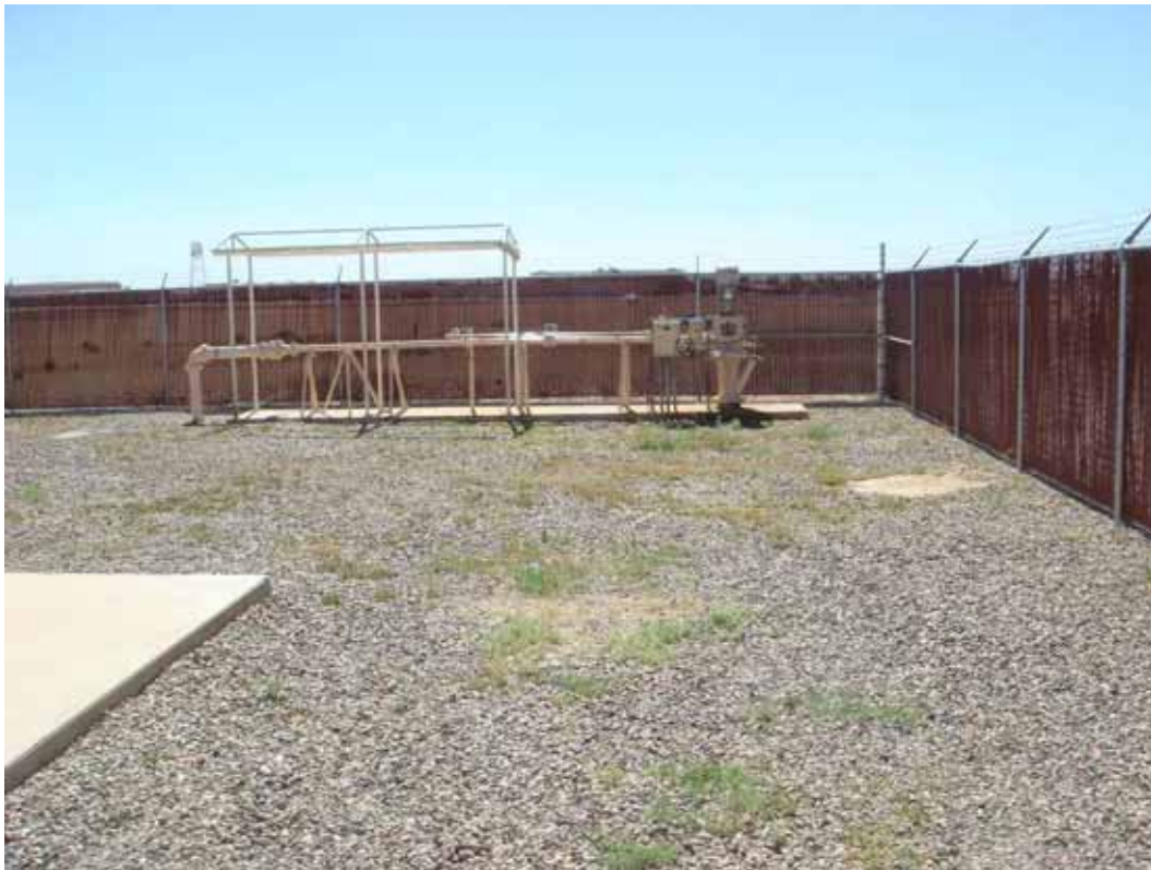
Photo 31. PGAS Site Visit. Subunit C extraction well (E-102).
