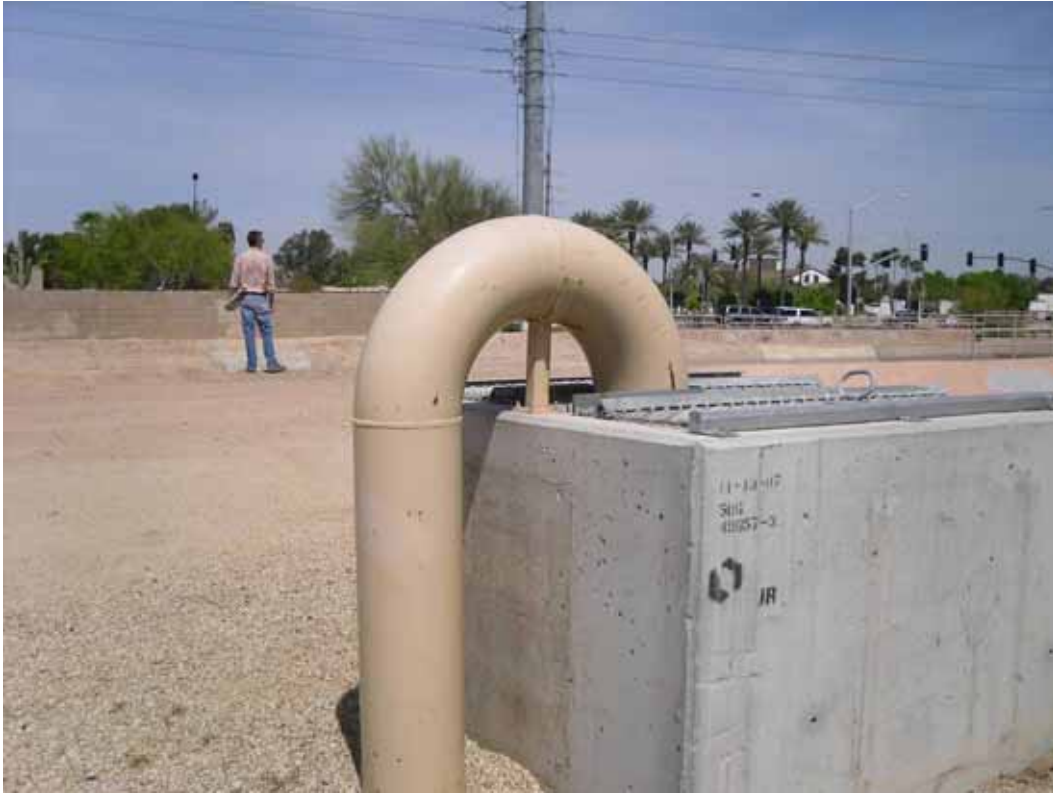
Photo 10. PGAN Site Visit. EA-06 treated effluent discharge.
