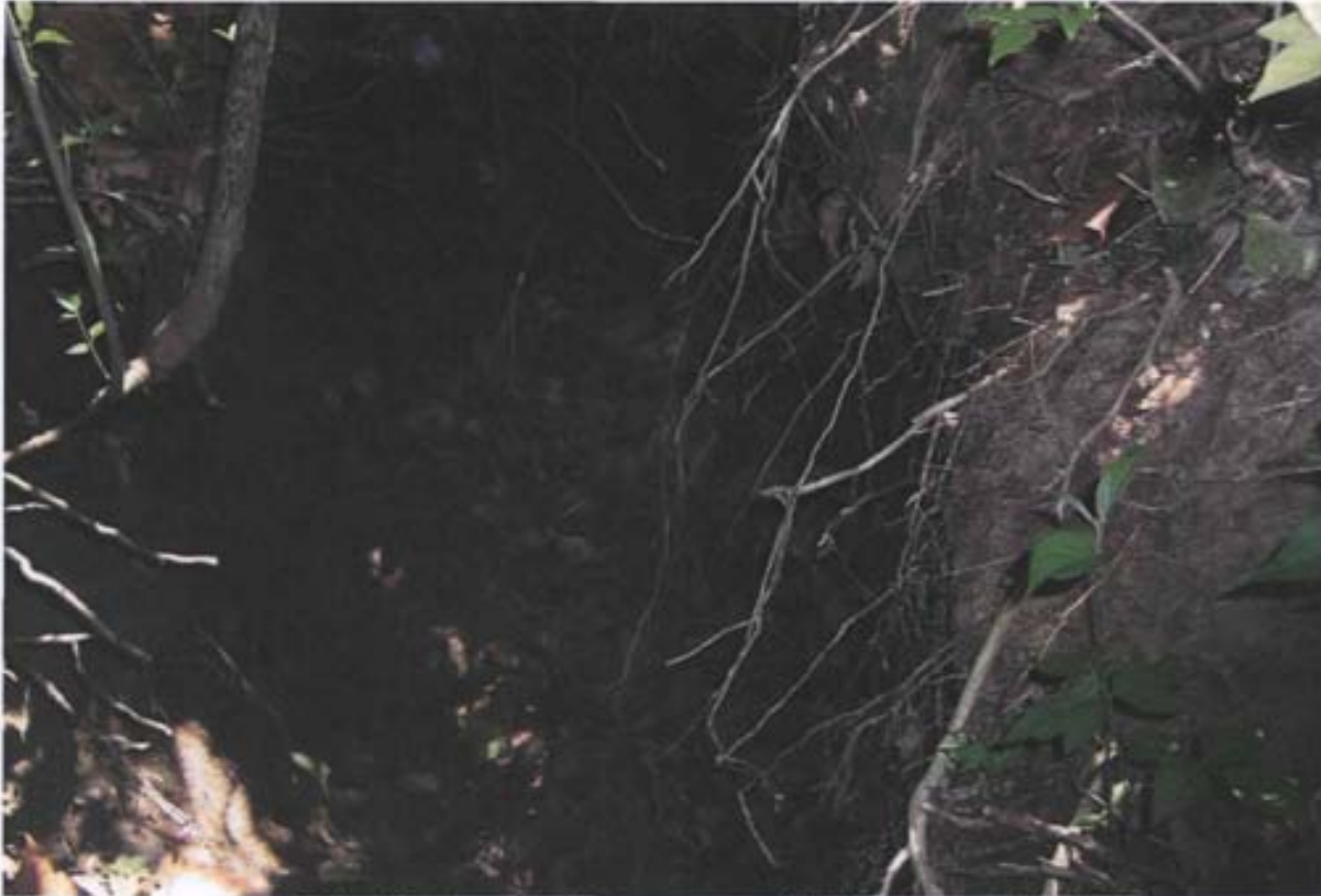
Photo 42: Close-up of 20 by 4-foot erosion feature near north IC boundary at Site LF-34.
