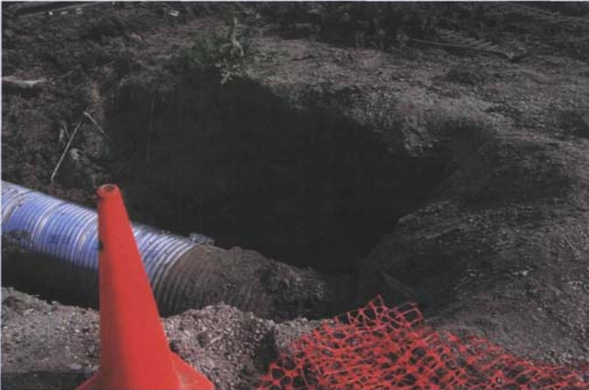
Photo 51: North view of roadway culvert replacement at Site LF-42.
