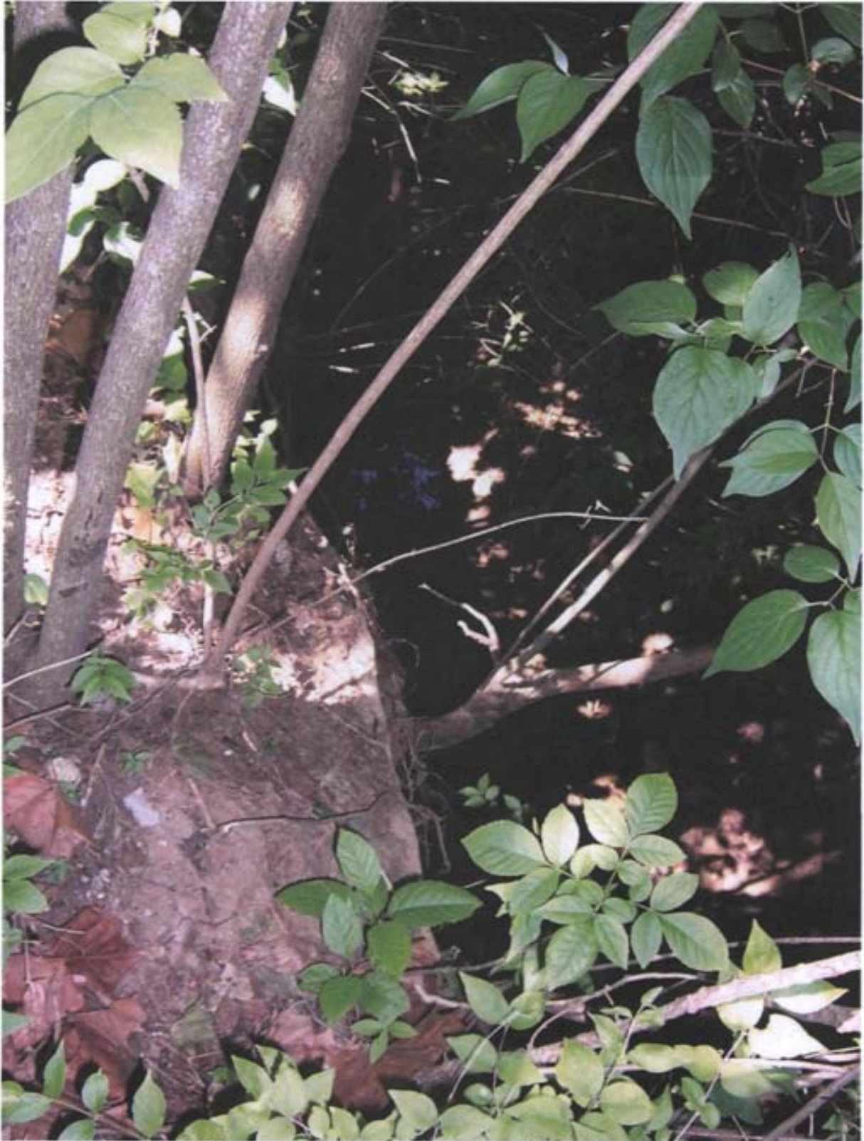
Photo 41: Close-up of 20 by 4-foot erosion feature near north IC boundary at Site LF-34.
