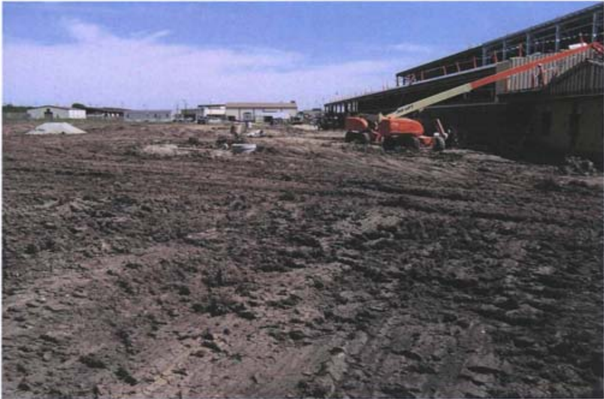
Photo 7: North view of west IC boundary of Site FT-02.
