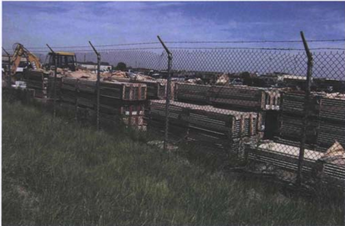
Photo 3: Northwest view of construction parking area and construction storage area at Sites FT-02, LF-12, and SS-44.
