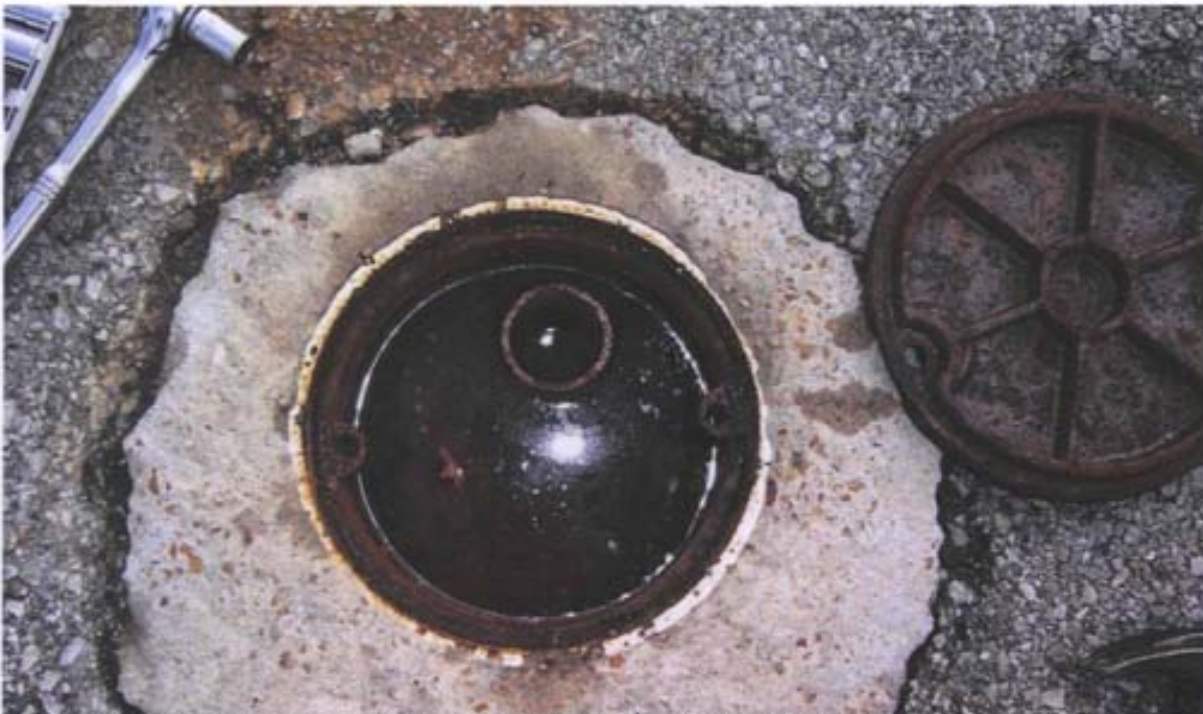
Photo 29: Close-up of partially submerged well protector at SS30-MW-19.
