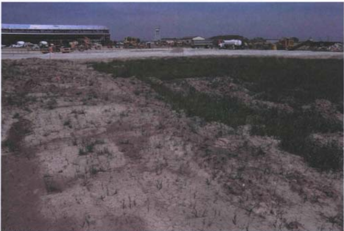
Photo 4: West view of construction activities at Sites FT-02, LF-12, and SS-44.
