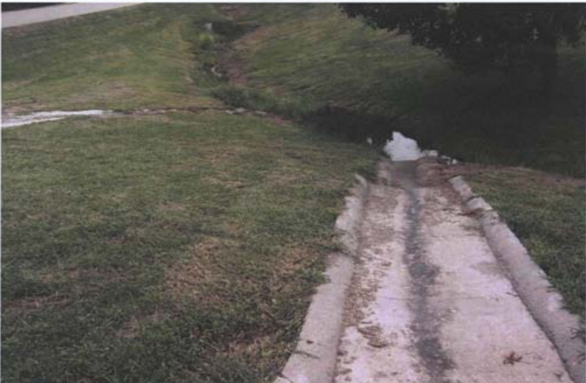
Photo 37: East view of surface water sample SS30-SW-01 location.
