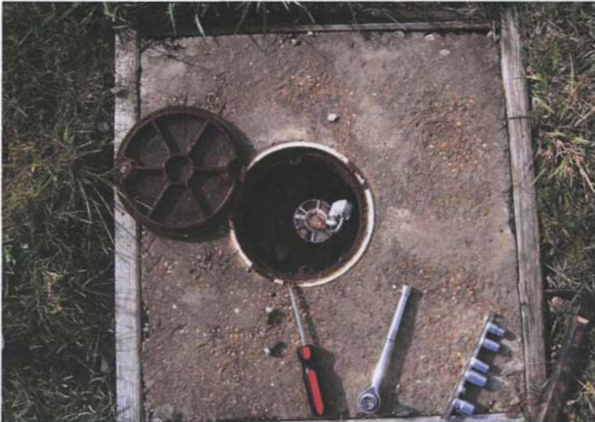
Photo 32: Close-up of monitoring well SS30-MW-20 at Site SS-30.
