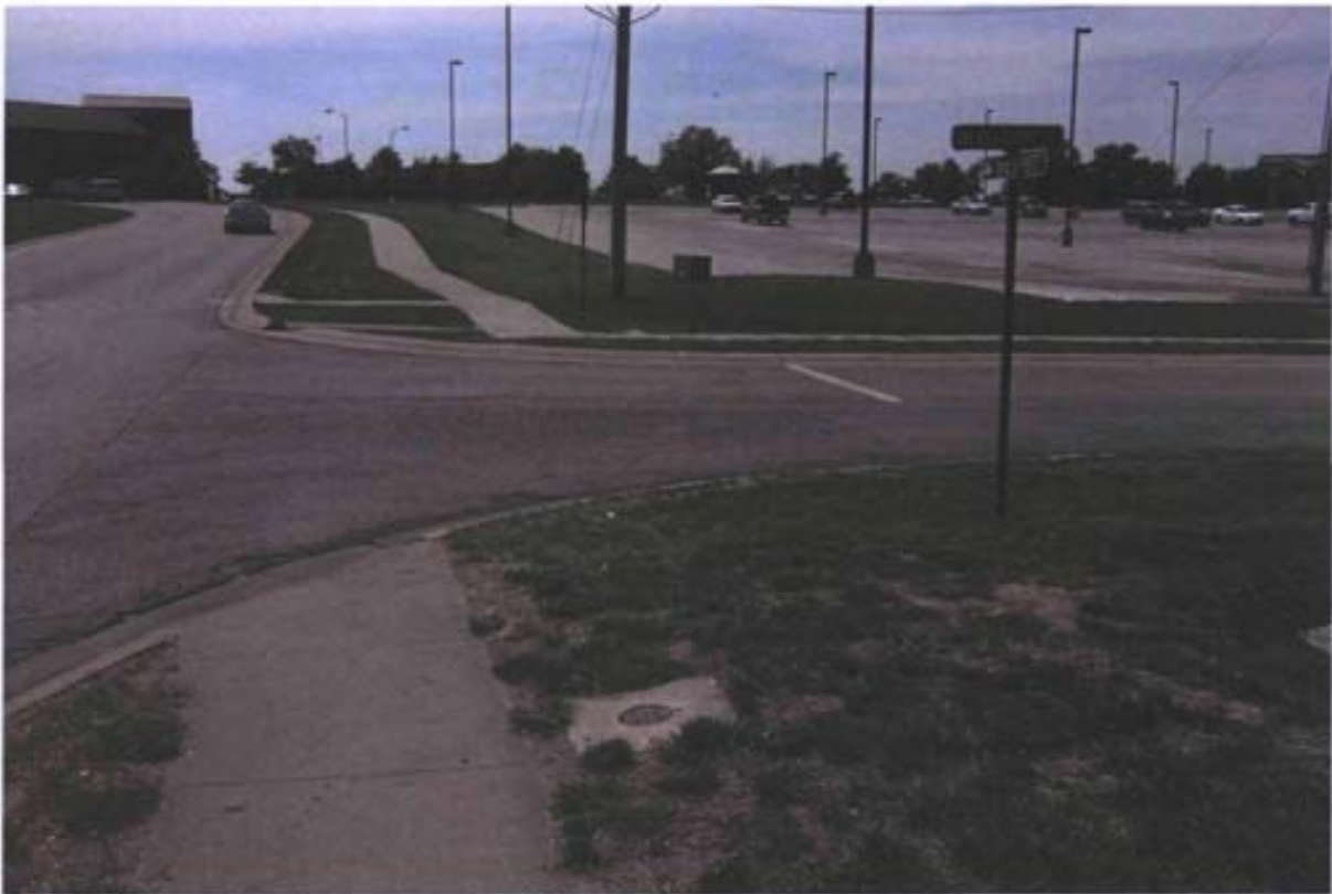
Photo 23: West view of central portion of Site SS-30.
