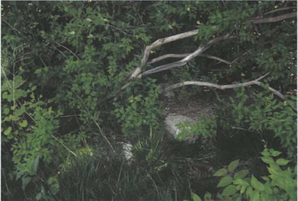
Photo 44: Northwest view of exposed concrete near west-northwest portion of Site LF-34.
