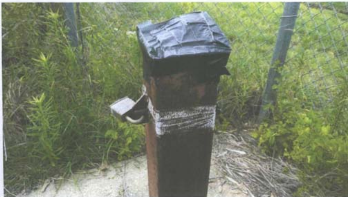
Photograph No. 29 Description: MW-30 detail of taped cover. Date: June 15, 2010
