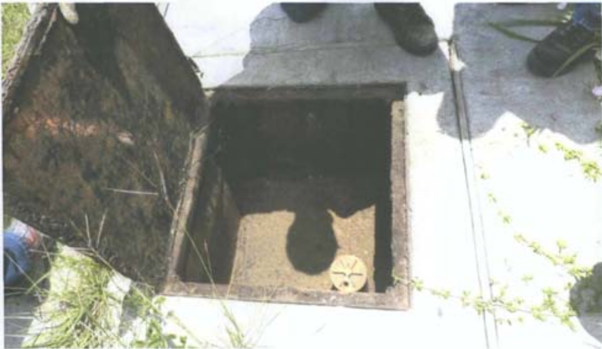
Photograph No. 43 Description: Monitoring well SW-1; cover was unlocked; inside view. Date: June 15, 2010
