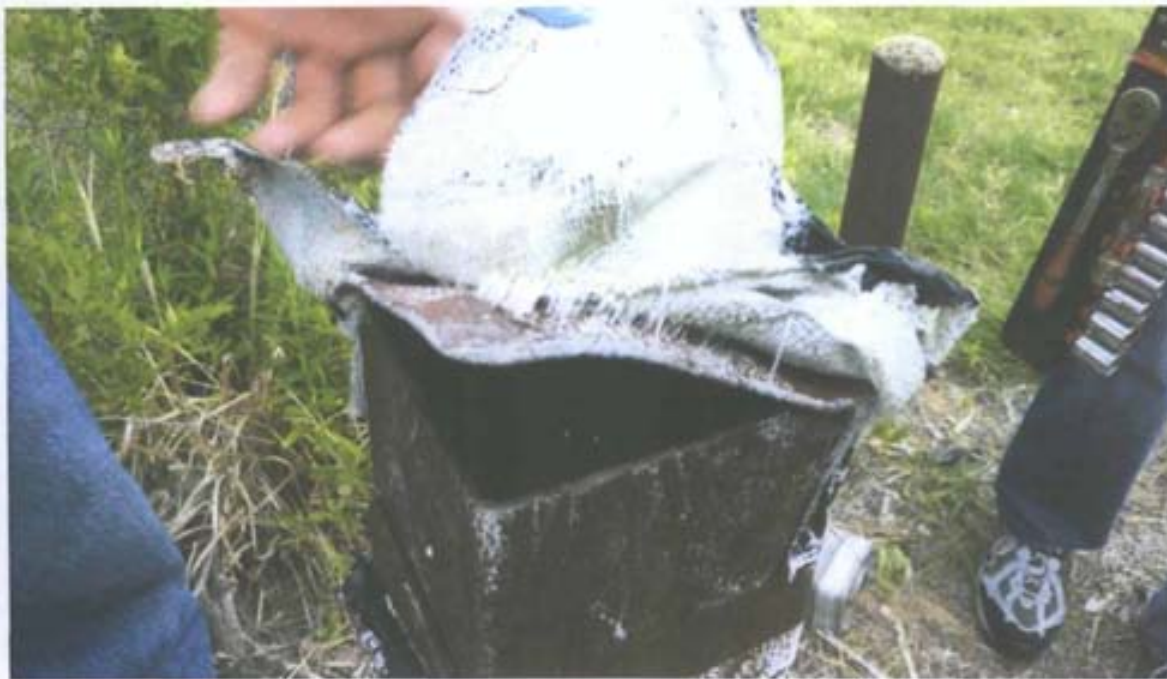
Photograph No. 30 Description: MW-30 detail with duct tape removed. Date: June 15, 2010
