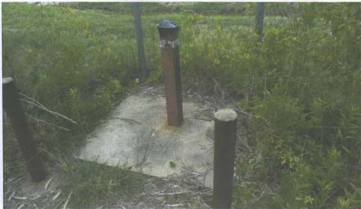
Photograph No. 28 Description: Well MW-30; metal protective casing cover is broken and was sealed with duct tape. Date: June 15, 2010
