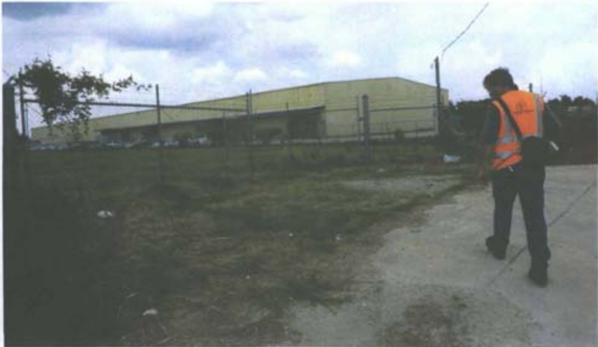
Photograph No. 78 Description: Entry to the Levy Tract; note no signage posted on fence. Date: June 15, 2010
