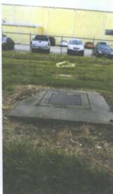
Photograph No. 80 Description: PRS well MW-SW-3; note electrical box for the PRS in background, marked by yellow tape during mowing. Date: June 15, 2010
