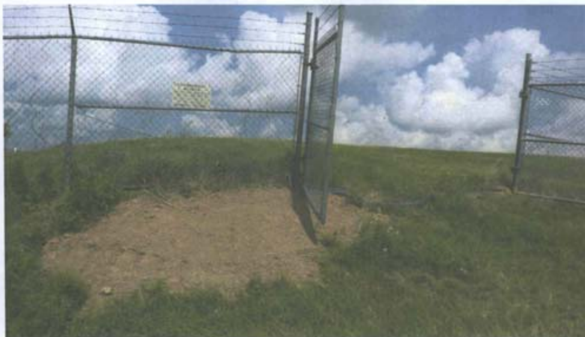
Photograph No. 1 Description: Southeast gate to monofill. Date: June 15, 2010
