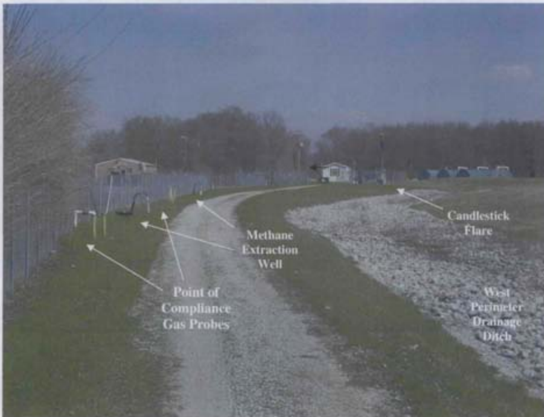
West perimeter road, drainage ditch, gas monitoring probes, methane extraction wells, and candlestick flare
