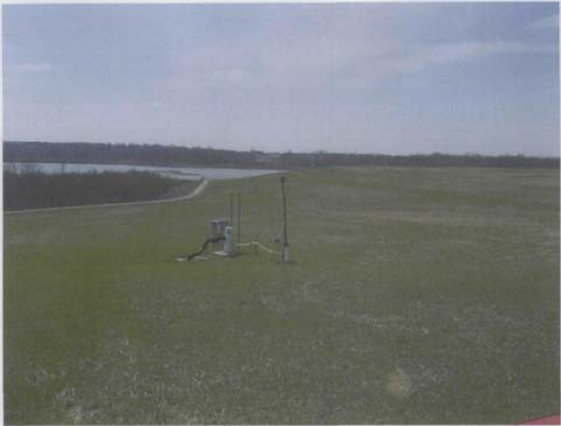
Landfill cover with vegetation and extraction well facing south-southwest towards old stone quarry
