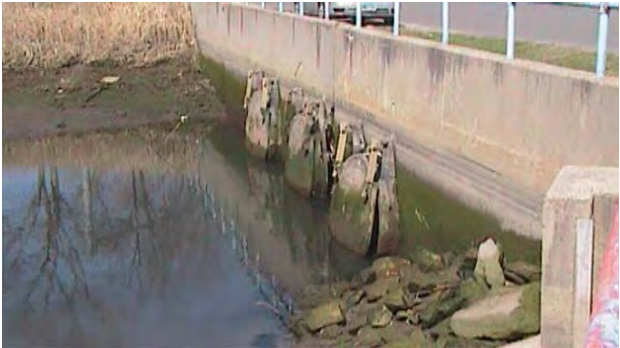
Ferry Creek flood gate.
