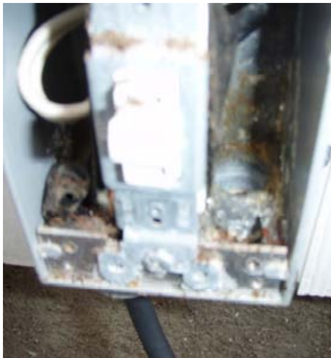
Photograph 12) House #27 – 232 Housatonic Avenue: Electric Box
