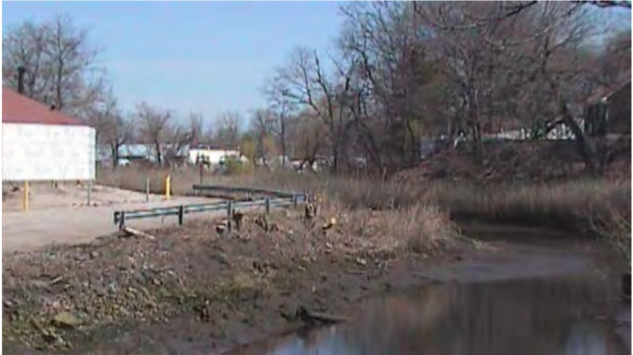
Ferry Creek looking upstream from the floodgate.
