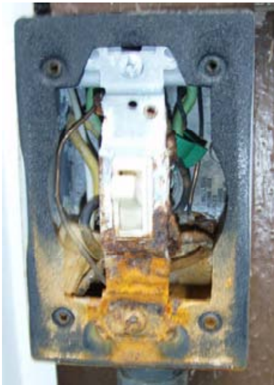
Photograph 13) House #46 – 405 Housatonic Avenue: Electric Box
