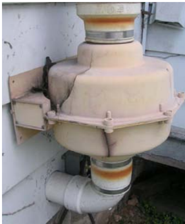
Photograph 10) House #25 – 125 Homestead Avenue: Fan Casing
