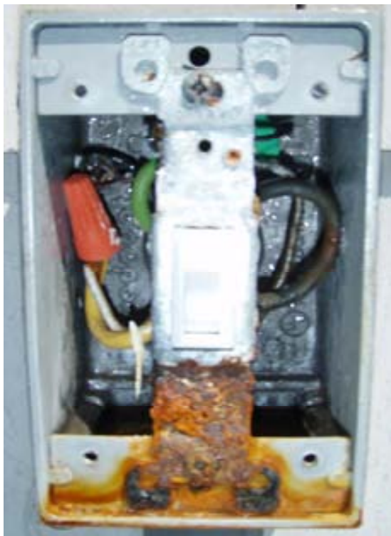
Photograph 14) House #55 – 492 Housatonic Avenue: Electric Box
