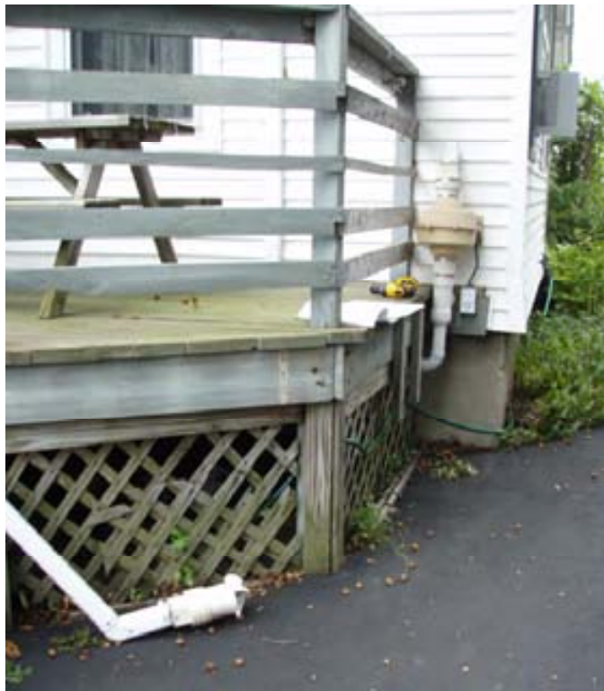
Photograph 11) House #26 – 231 Housatonic Avenue: Vent Pipe and Cap
