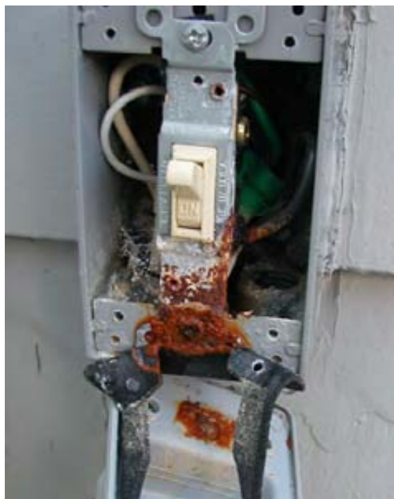
Photograph 16) House #67 – 56 Minor Avenue: Electric Box
