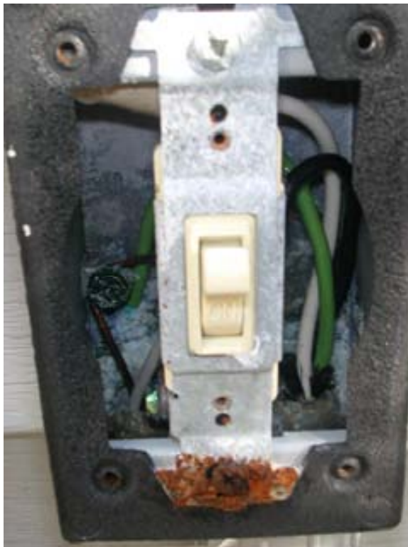
Photograph 15) House #62 – 560 Housatonic Avenue: Electric Box
