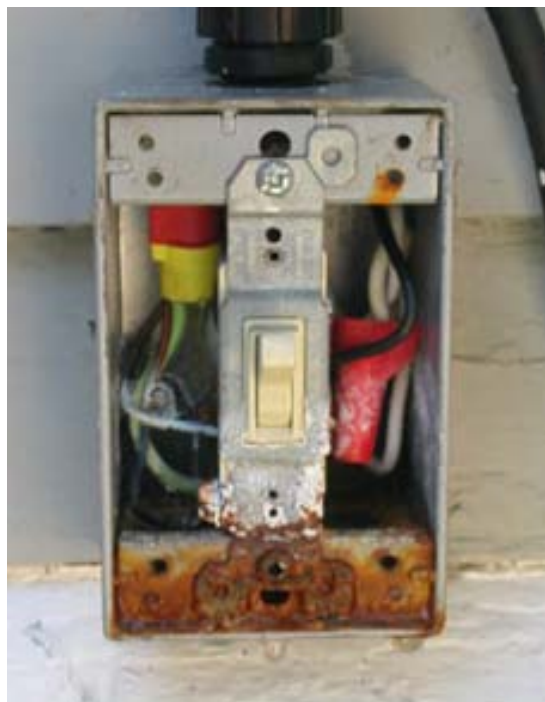
Photograph 18) House #70 – 83 Minor Avenue: Electric Box
