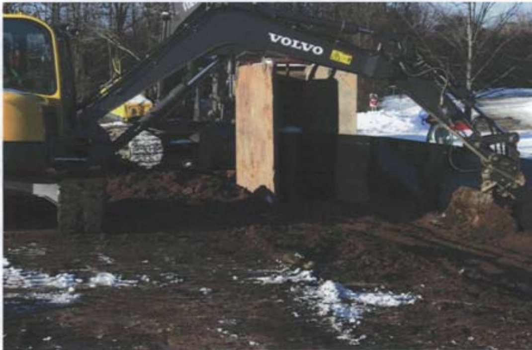
Photo Number 5 – December 2009: Installation of vertical landfill barrier.
