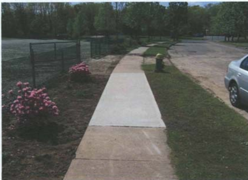
Photo Number 7 – April 2010: Repaved sidewalk after restoration work from winter activities. View to the west.
