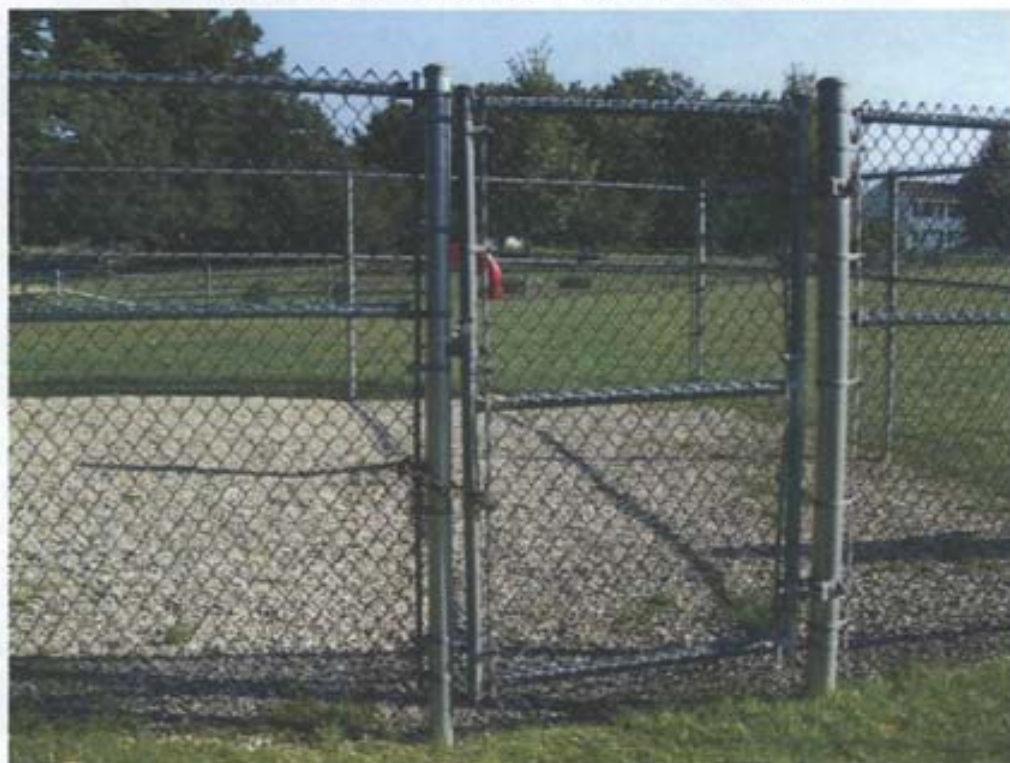
Photo Number 10 – Gas Vent (GV-1) secured with fencing
