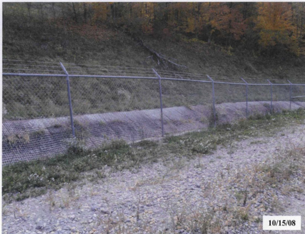
Kings Run lined outside of fence, facing southeast
