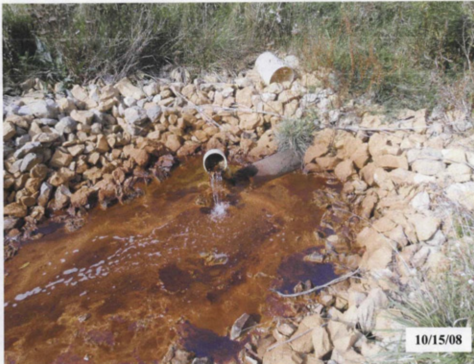
French drain transported collected groundwater and leachate to the Southern Toe.
