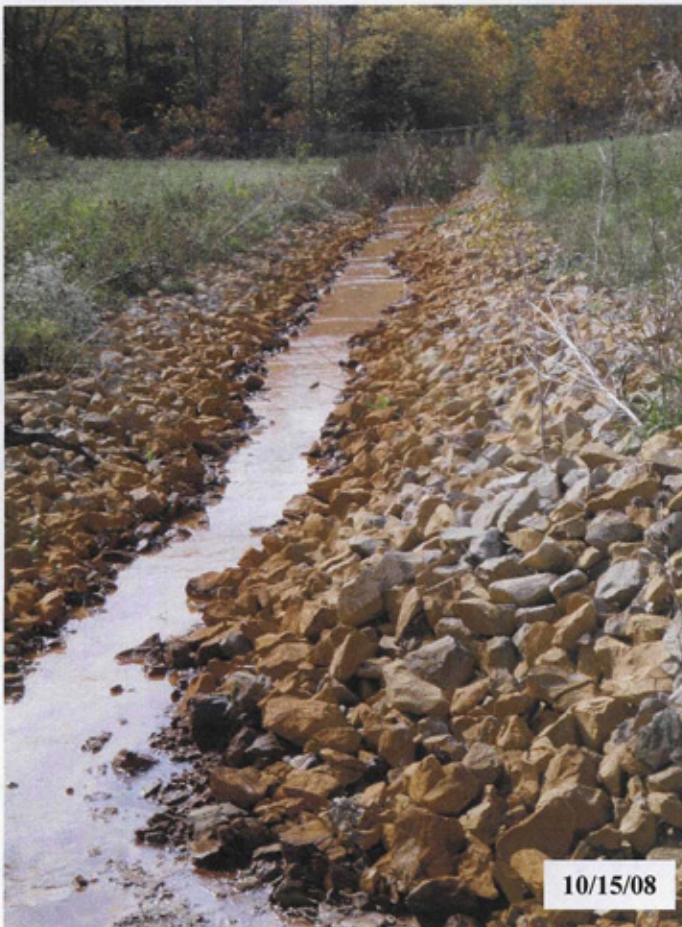
French drain transported collected groundwater and leachate to the Southern Toe.
