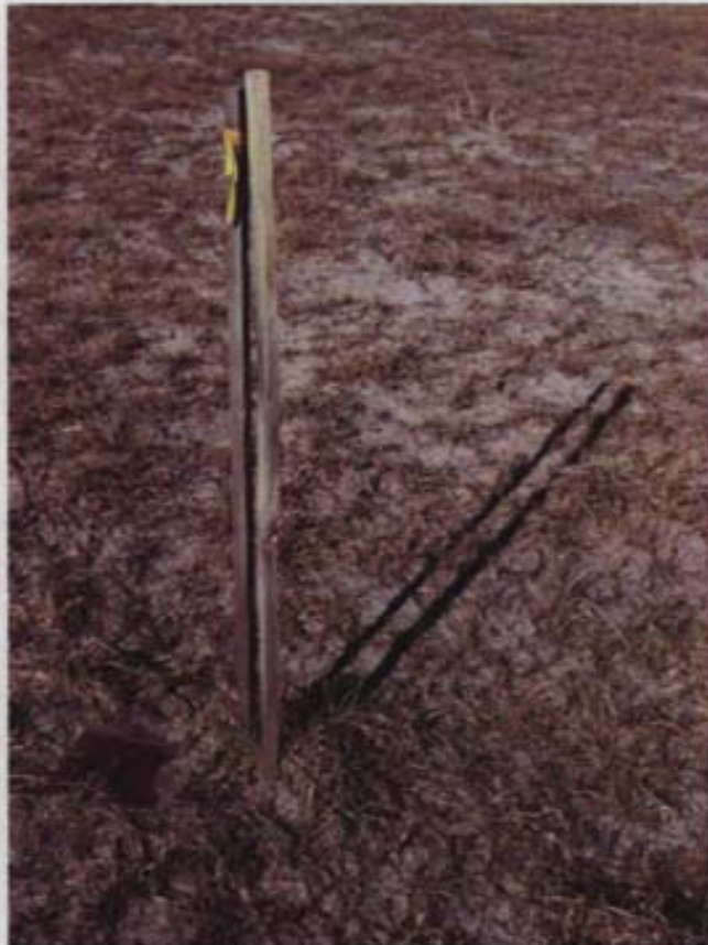
Marked settlement monument used to monitor the soil cover.
