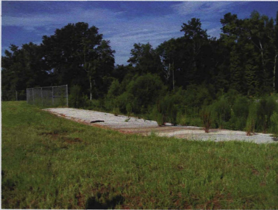
Fence opening for the drainage area where trespassers can enter the Site.
