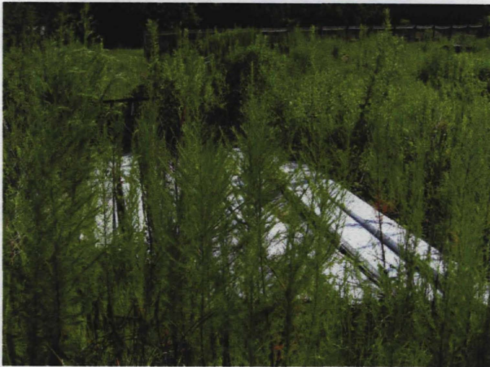
Debris located outside of the fence surrounding the cap on the northeast corner of the Site.
