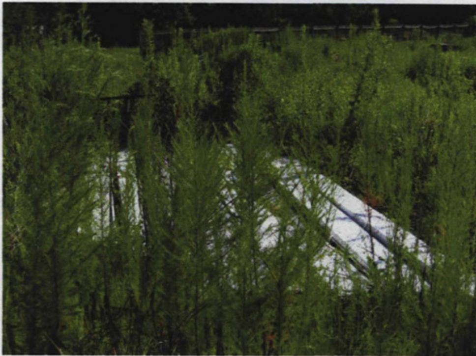
Debris located outside of the fence surrounding the cap on the northeast corner of the Site.
