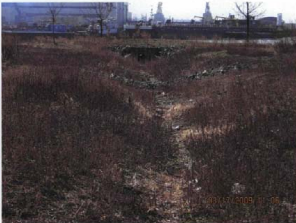
DRAINAGE SWALE IN AREA A
