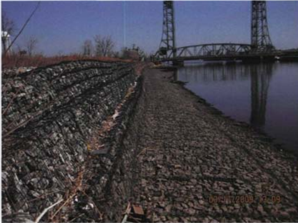
VIEW OF GABION BASKETS TOWARD LIFT BRIDGE
