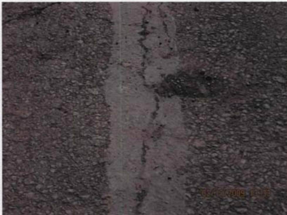
AREA B CAP SHOWING CRACK REPAIR
