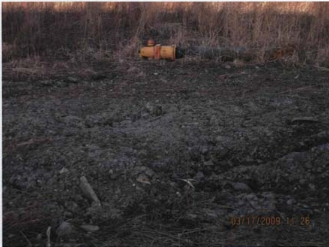
EXCAVATION FROM WATER LINE CAPPING PROJECT
