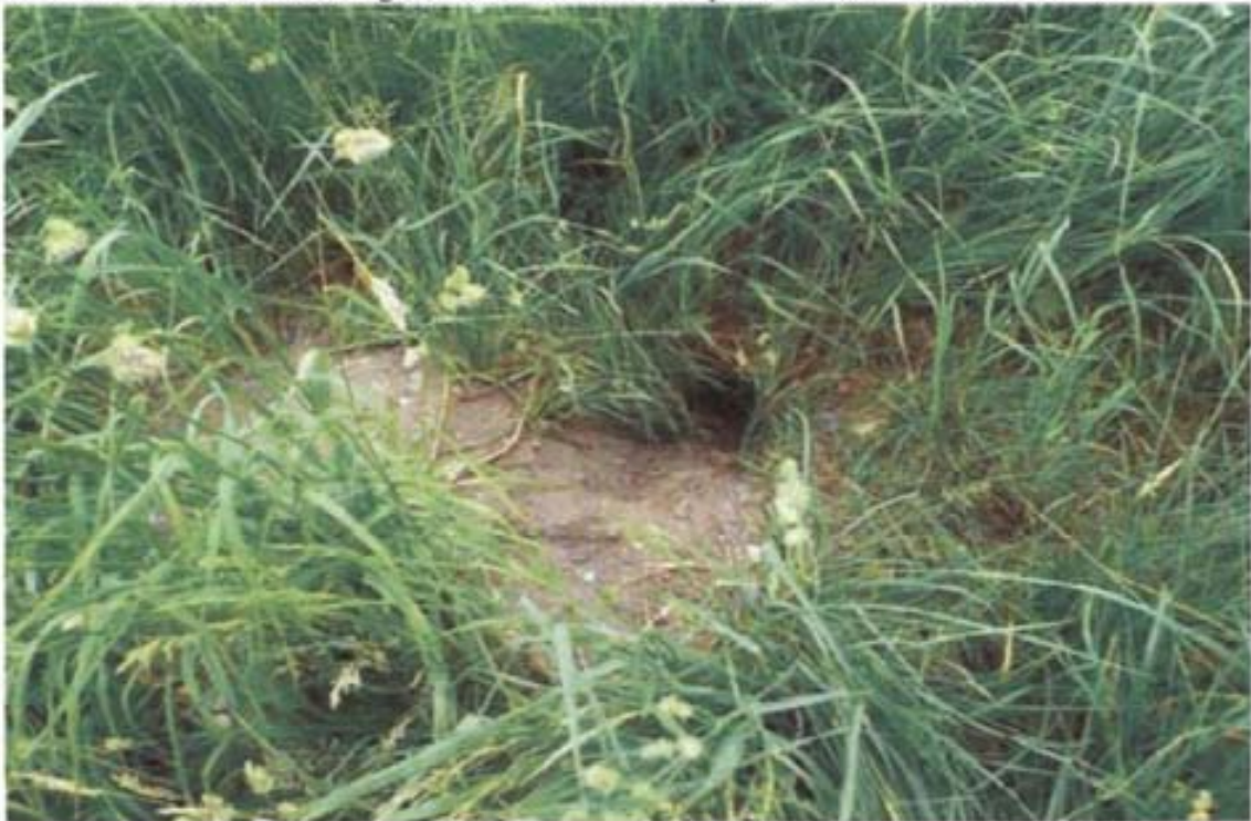
Photo 8 Animal burrow at edge of land fill crest at mid-point between GV-4 and GV-5.
