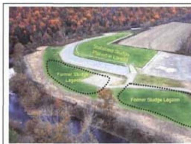
Post-remediation view of lagoon area
