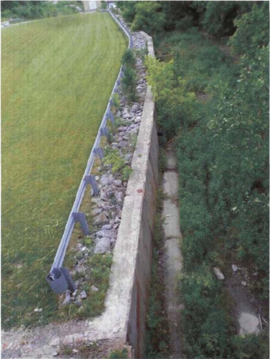
Photo 23 Retaining wall appears structurally sound and stable.
