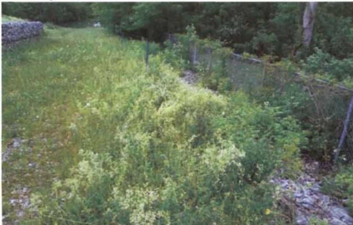
Photo 20 Large trees and bushes should be cleared at least 3 ft from either side of fence.
