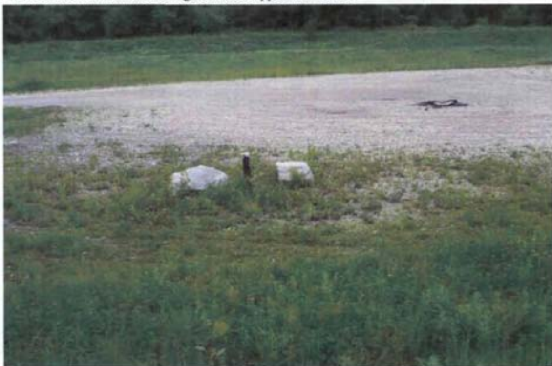
Photo 6 Groundwater monitoring wells are capped and locked.
