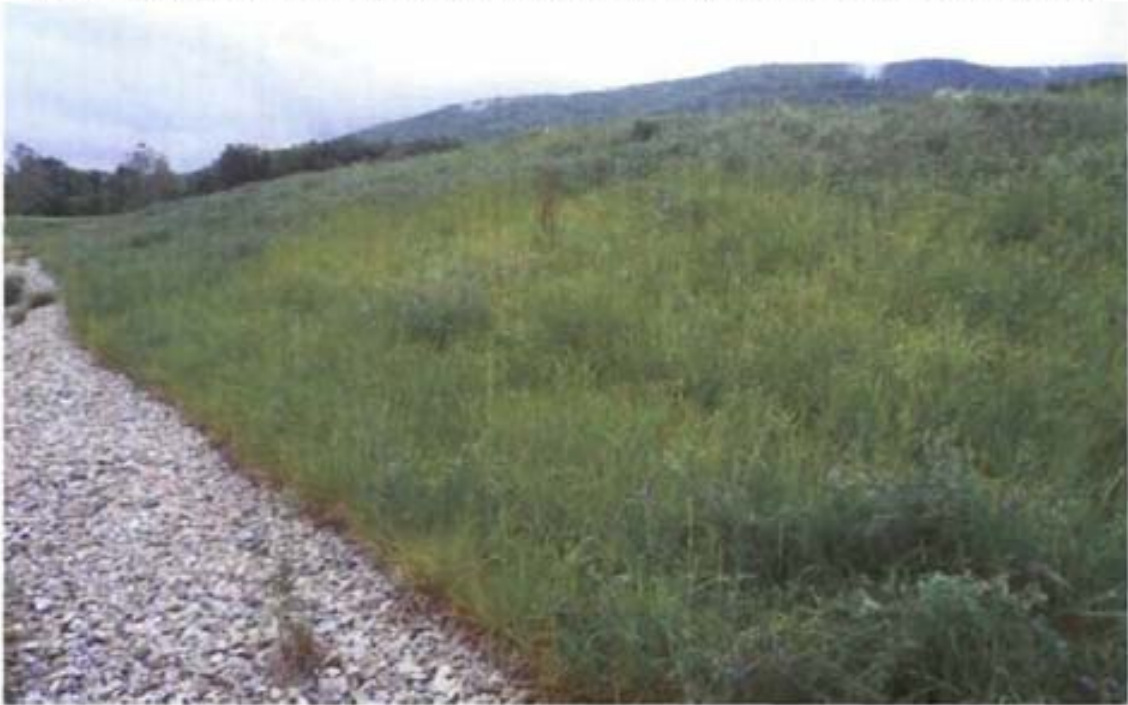
Photo 1 No signs of instability or erosion on side slopes. Landfill side slopes need mowing.
