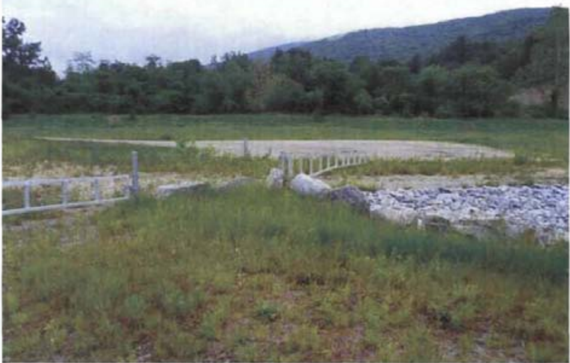
Photo 10 Gravel road requires maintenance. Perimeter fence is in good condition.
