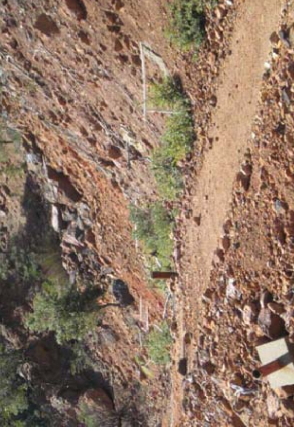
PVC horizontal drains in Boulder Creek landslide area. The exposed PVC piping should be coated or replaced with UV-resistant piping.
