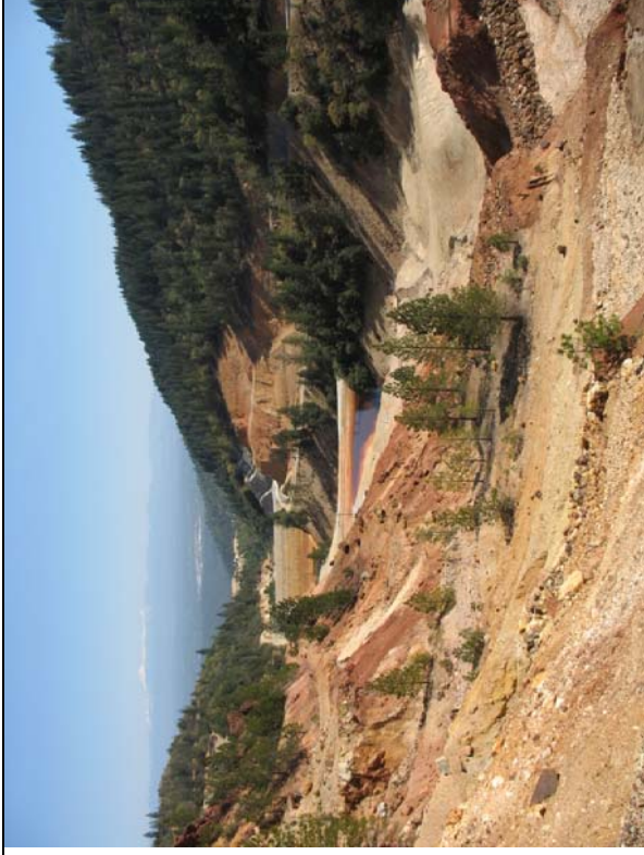
SCRR sedimentation basin and rock check dams, looking east. The rock check dams are performing well.
