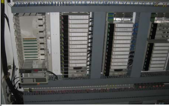
MFTP Control Center. Programmable logic controller (PLC) system updated in September 2007.
