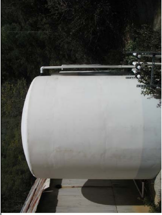
Three 6,500-gallon poly tanks are on the east side of the shed. Per IMO discussion with Ted Arman, the tanks contain raw Acid Mine Drainage, Sodium Silicate, and Ag-Gel fertilizer product.
