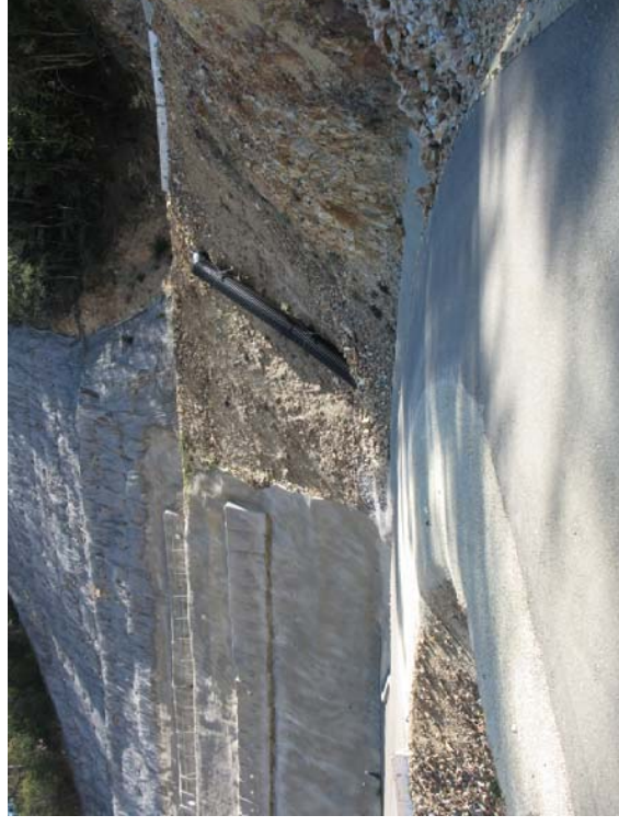
SCRR sedimentation basin and rock check dams, looking east. The rock check dams are performing well.
