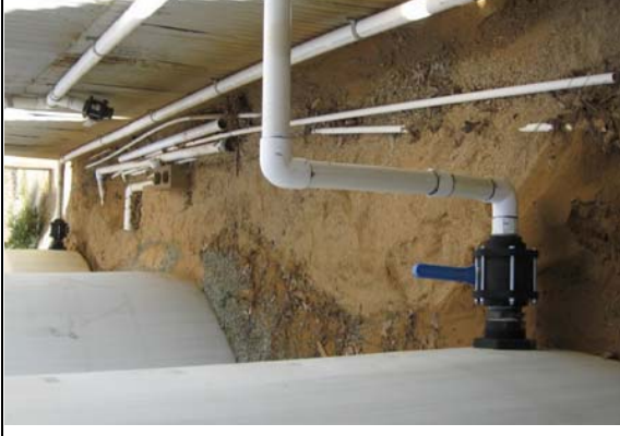
Three 6,500-gallon poly tanks are on the east side of the shed. Per IMO discussion with Ted Arman, the tanks contain raw Acid Mine Drainage, Sodium Silicate, and Ag-Gel fertilizer product.
