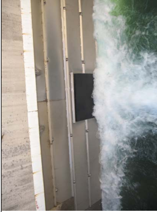
Upper Spring Creek Diversion Impact Structure. Stainless steel plates were installed during the 2004 annual maintenance event.
