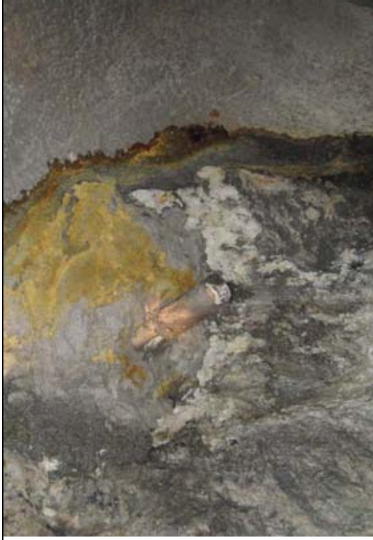
On 12/18/07, a leak of the AMD pipeline occurred near Road Marker 16.5 near the intersection of the AMD pipeline and the filtrate pipeline that extends from the Mine Waste Disposal Cell. Pipeline was repaired.
