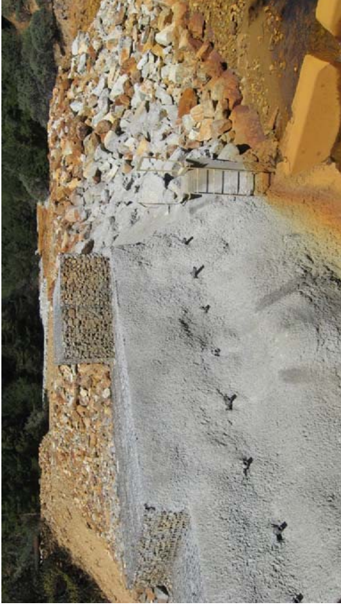
Boulder Creek Tailings Dam. Improvements were completed in 2005 to raise the dam, build the spillway, and improve Boulder Creek upstream.
